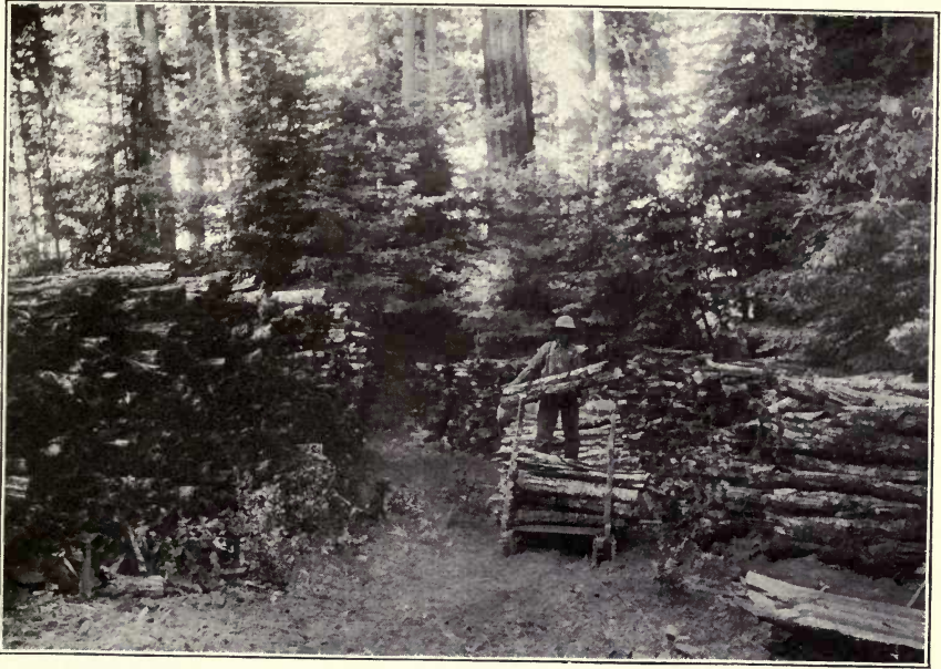
FIG. 1.—THE SKIDWAYS TO WHICH THE BUNCHED BARK IS SLEDDED, AND FROM WHICH IT IS HAULED TO THE RAILROAD.
