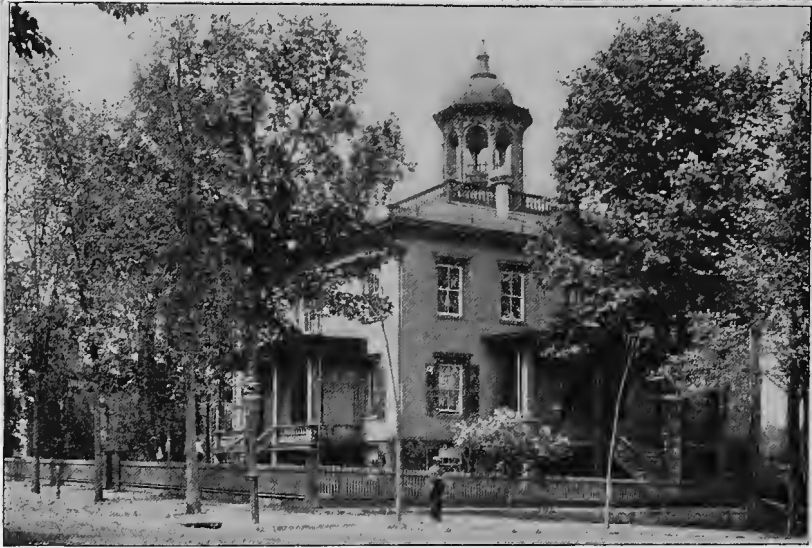
OLD COURT HOUSE.
