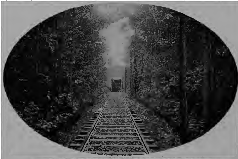
EASTERN NEW YORK RAILROAD, MILTON.
