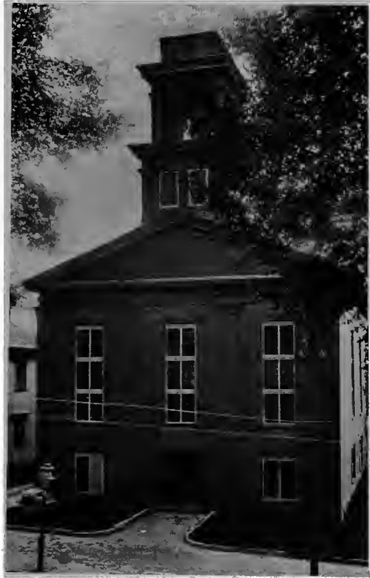
Methodist Church erected in 1845.
