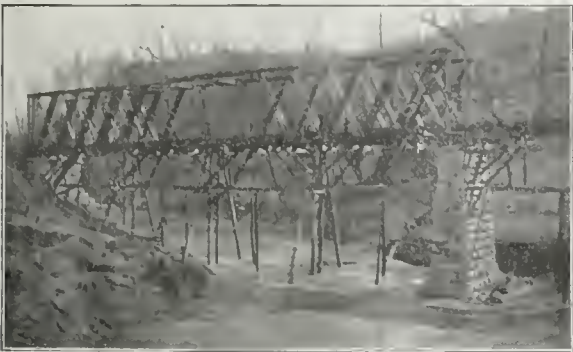
N., C. & ST. L. RAILWAY BRIDGE ACROSS CHATTANOOGA CREEK.
