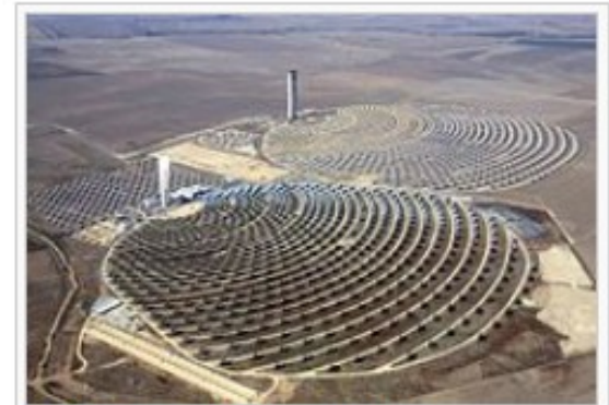
Solar power towers utilize the natural resource of the Sun, and are a renewable energy source. From left: PS10 and PS20 solar towers.
