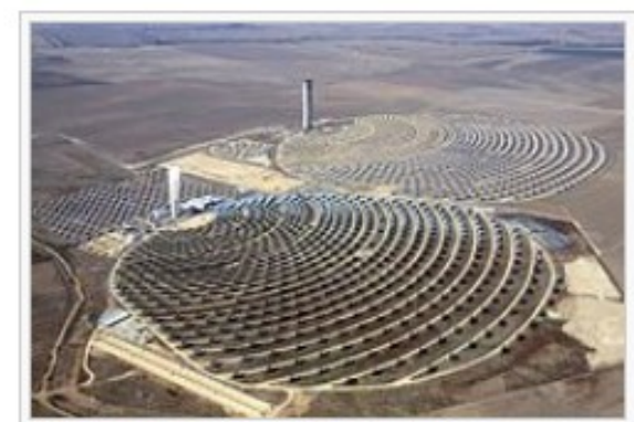
Solar power towers utilize the natural resource of the Sun, and are a renewable energy source. From left: PS10 and PS20 solar towers.
