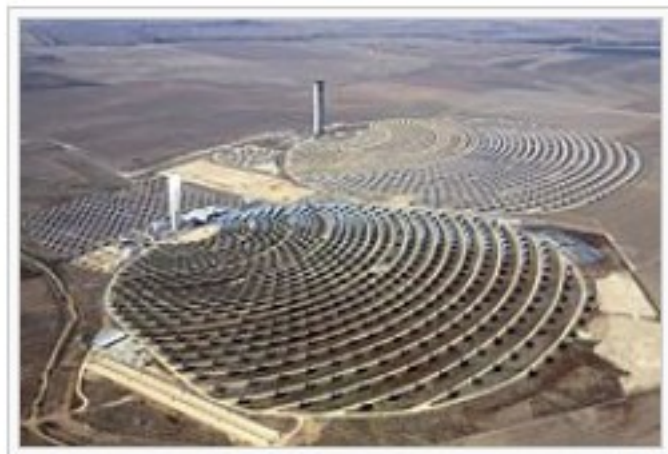
Solar power towers utilize the natural resource of the Sun, and are a renewable energy source. From left: PS10 and PS20 solar towers.
