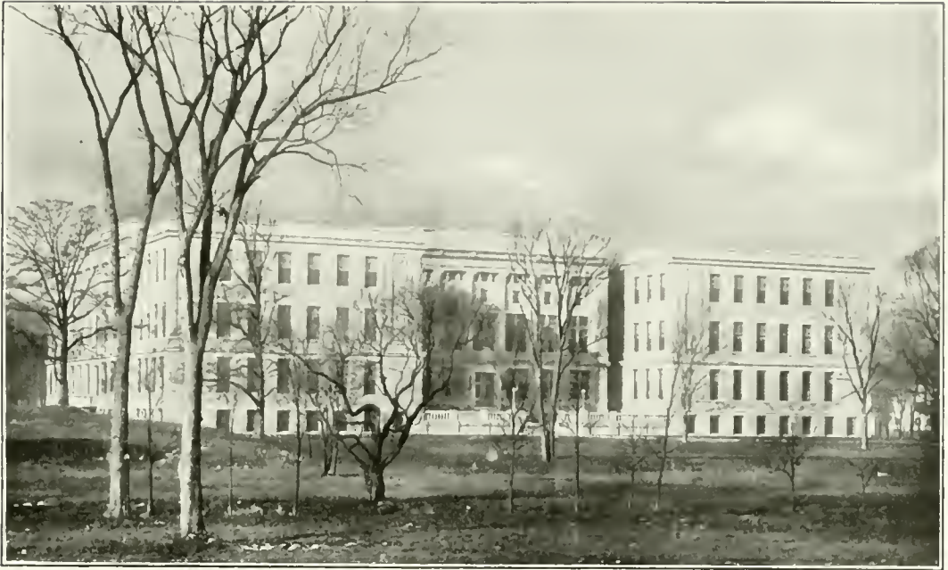
TECHNICAL HIGH SCHOOL, NEWTON, MASS. Geo. E. Newton, Architect
