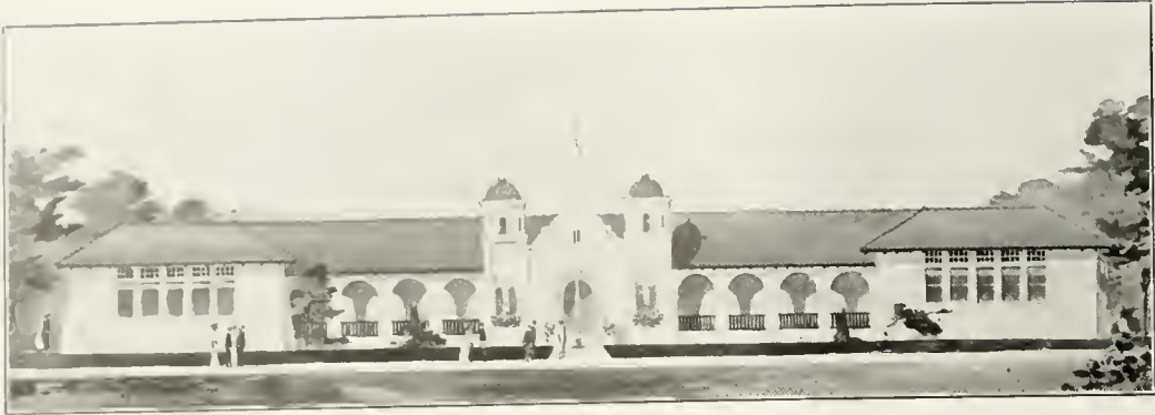
UNION HIGH SCHOOL, LINCOLN, CAL. Charles H. Parker, Architect, San Francisco, Cal.
