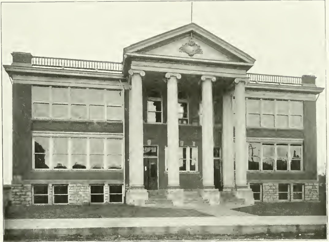
ALLEGHENY COUNTY HIGH SCHOOL, CUMBERLAND, MD. Geo. F. Sansbury, Architect, Cumberland
