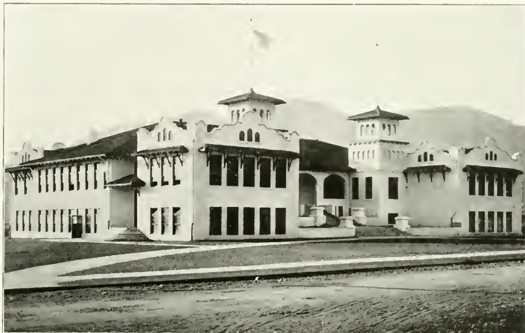
FILLMORE UNION HIGH SCHOOL, FILLMORE, CAL. A. C. Smith, Architect, Los Angeles, Cal.
