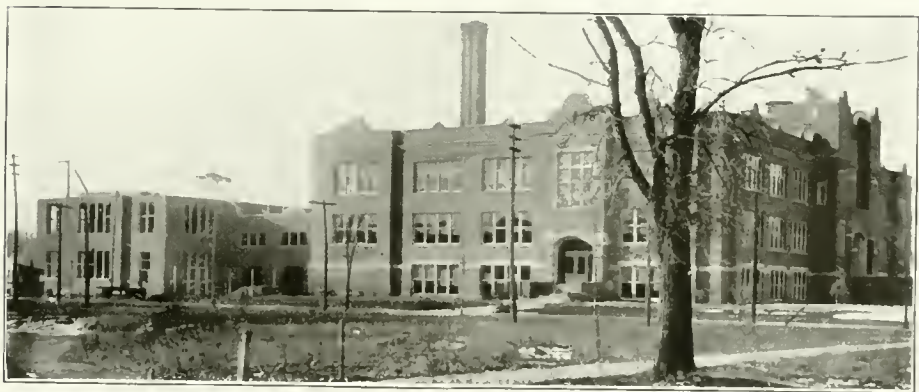
SIDE VIEW, LA CROSSE HIGH SCHOOL (Manual Training Addition under Construction)
