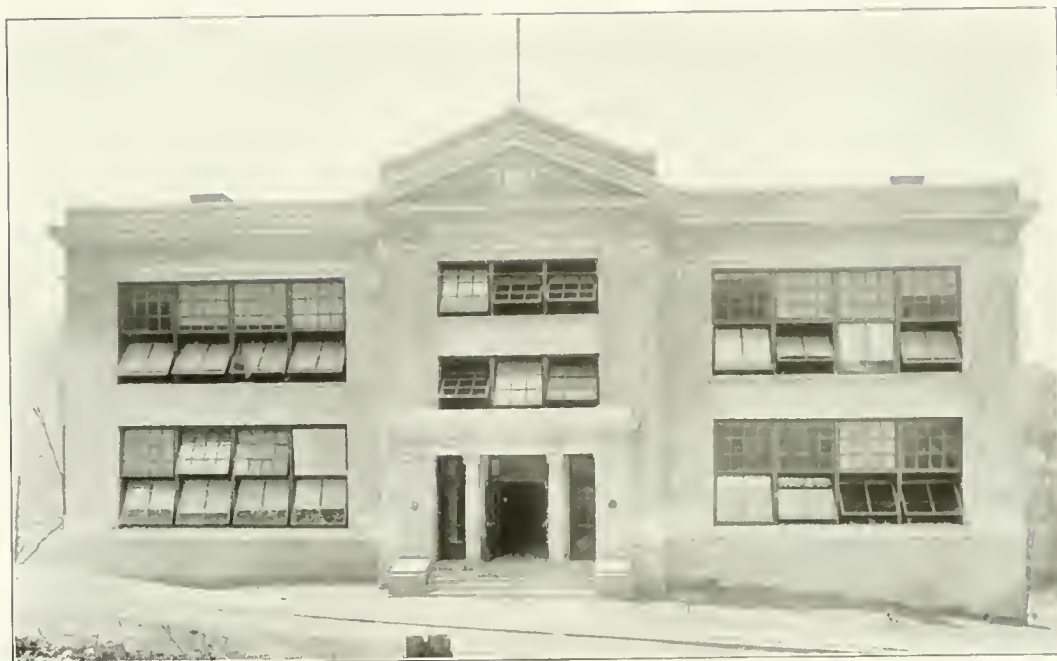
HIGH SCHOOL, WOODLAWN, PA. C. C. & A. L. Thayer, Architects, New Castle, Pa.
