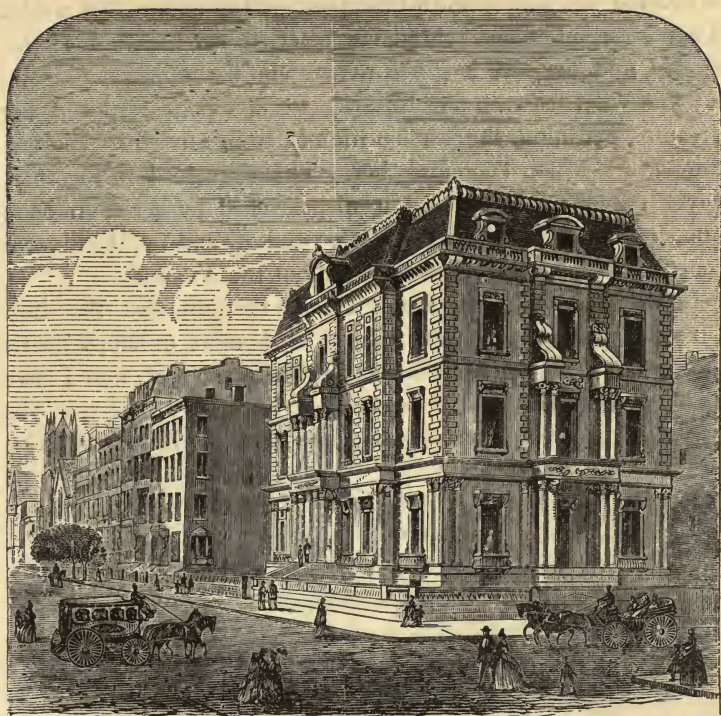
JUNCTION OF THE FIFTH AVENUE AND THIRTY-FOURTH STREET, SHOWING THE NEW RESIDENCE OF A. T. STEWART, ESQ.
