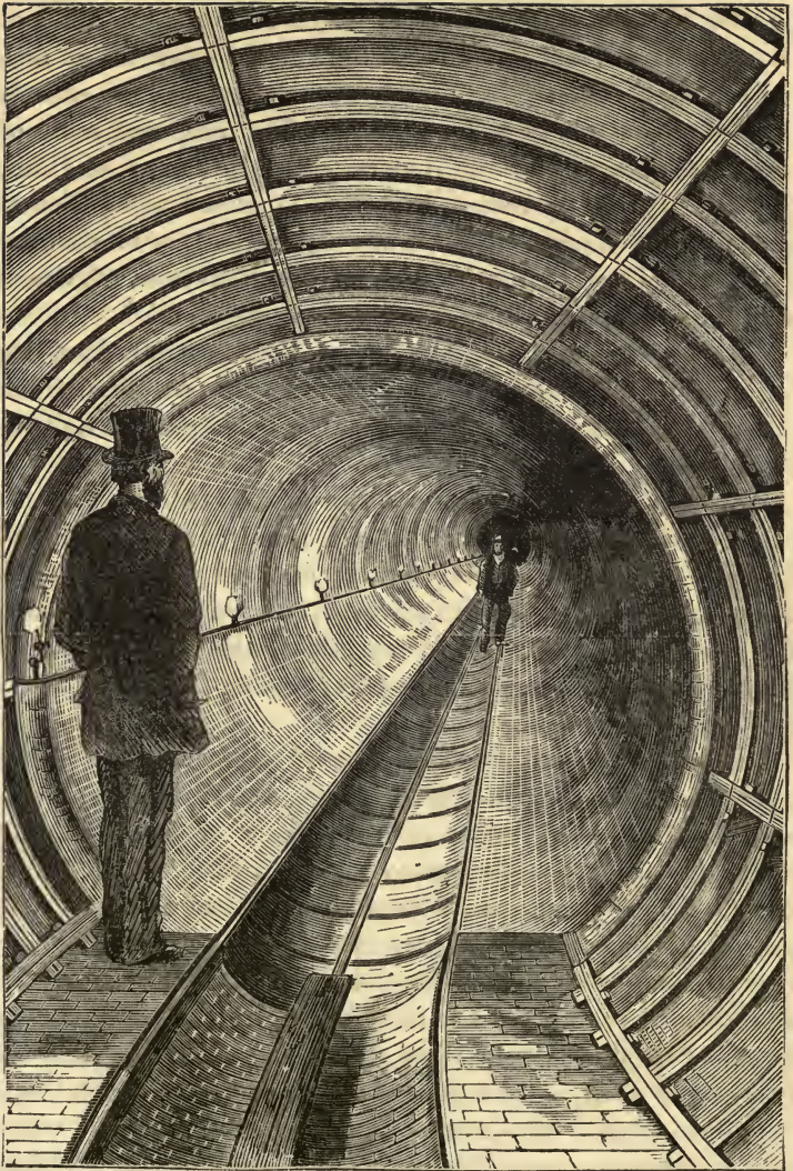
TUNNEL UNDER BROADWAY.
