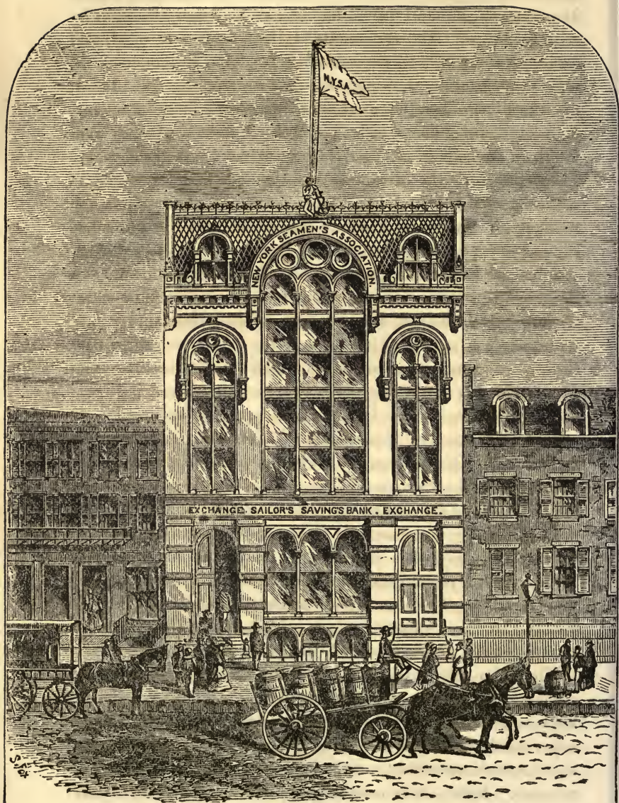
NEW YORK SEAMEN'S EXCHANGE BUILDING.
