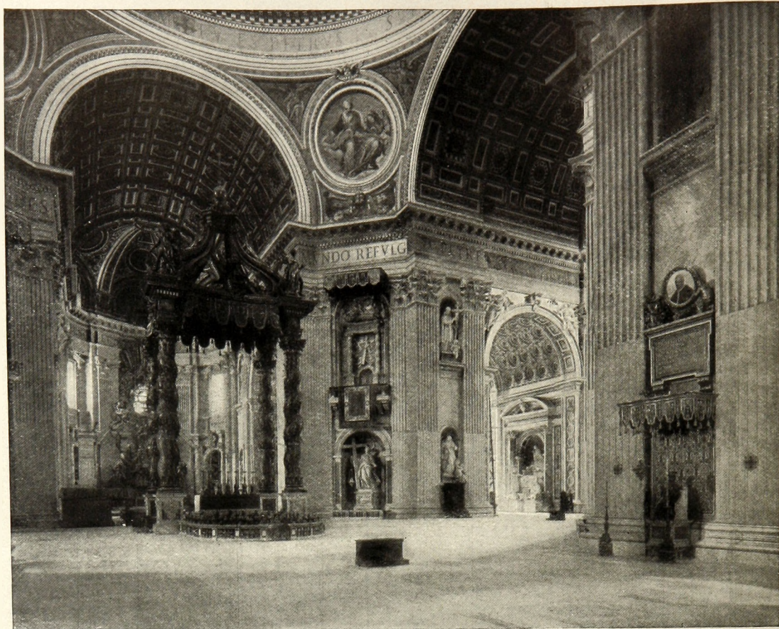
INTERIOR COURT OF SAINT PETERS
