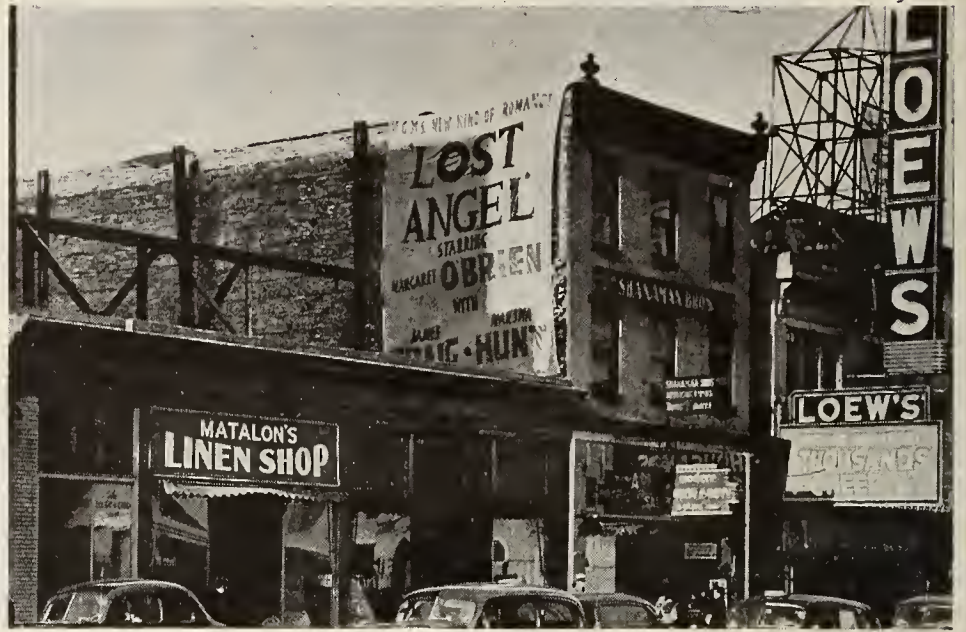
Manager Sam Gilman, of Loew's Regent, Harrisburg, Pa., took advantage of an adjoining building being demolished and spotted this huge banner where townspeople couldn't miss seeing it.
