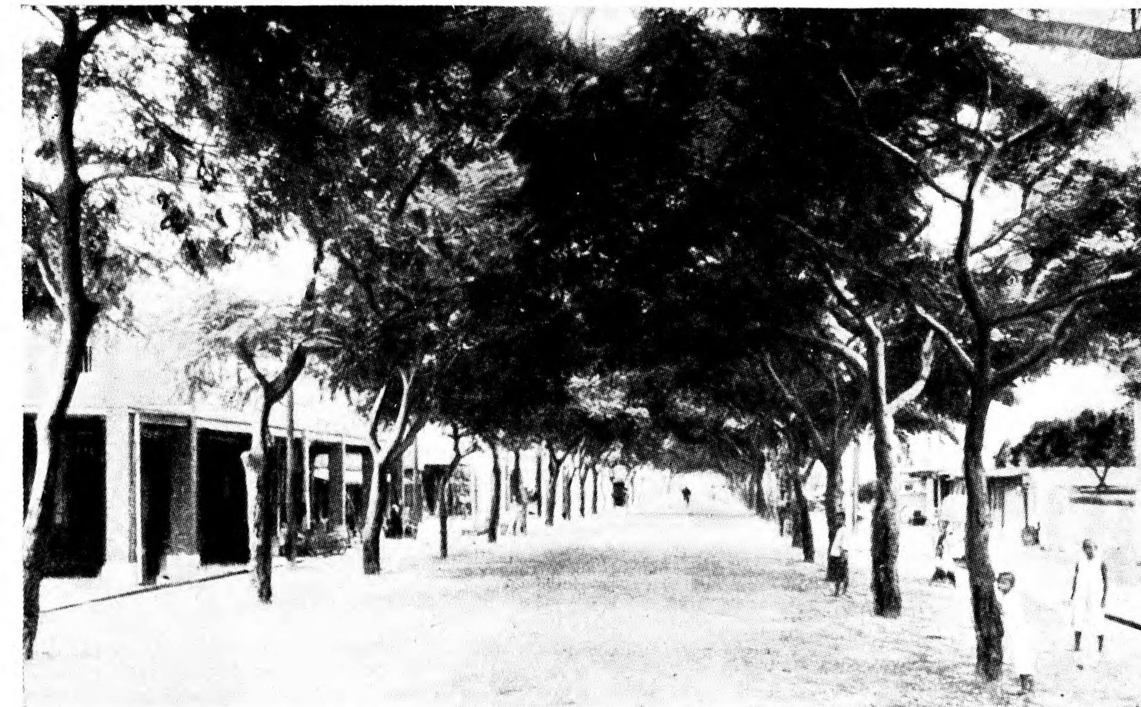
17. Rebuilt street in Tainan City, from main railway station to provincial government buildings.
