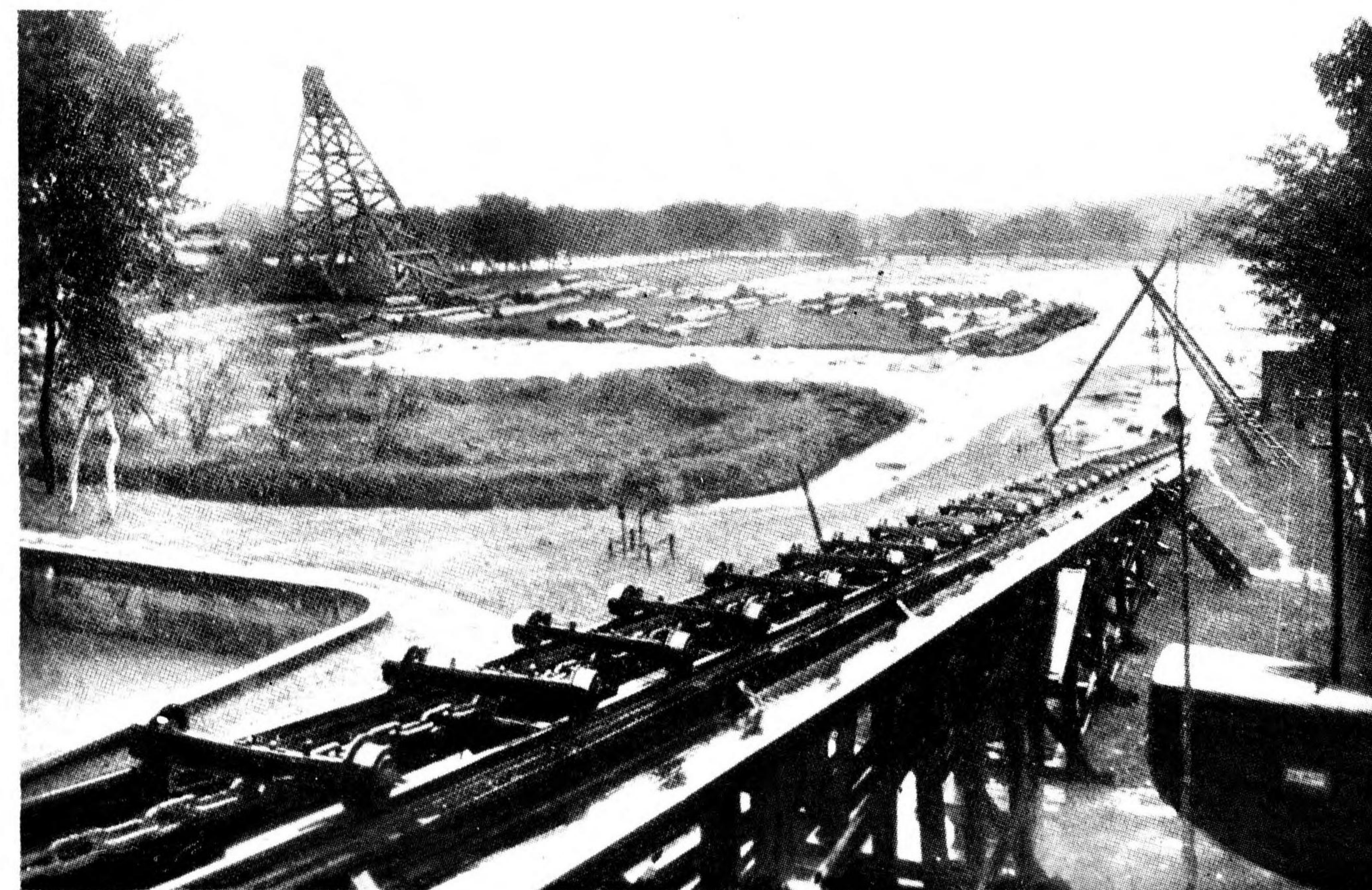
6. Logs being pulled out of the storage pond into the Kagi sawmill, said to be the largest in the Far East.
