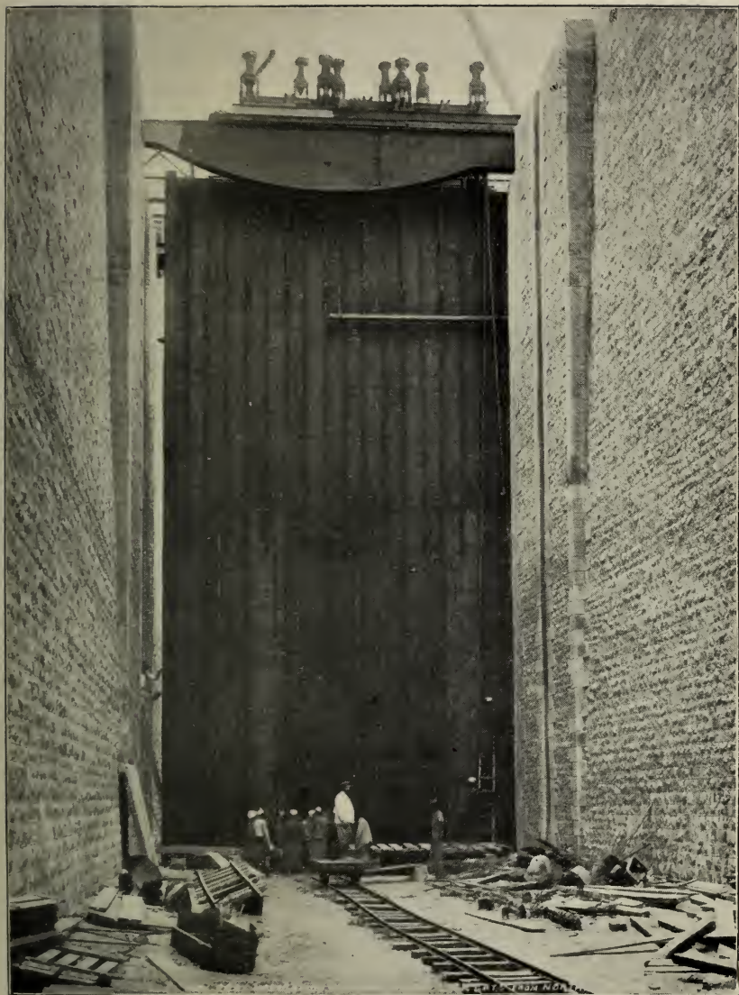
FIG. 6.—NAVIGATION CHANNEL: FIRST LOCK-GATE FROM NORTH.
