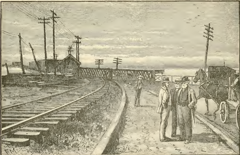
ENTRANCE TO LONG BRIDGE.
