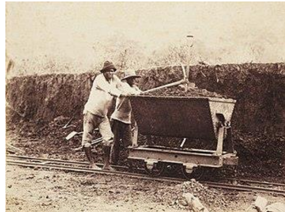
Jamaican canal construction workers in Panama, 1881-1889. Their V-skip wagons still have no locking system and a rectangular chassis instead of the subsequently used curved U-profiles.
