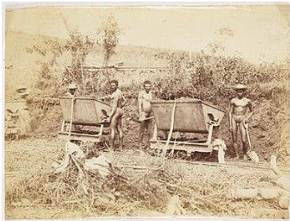
Jamaican canal construction workers in Panama, 1881-1889. Their V-skip wagons still have no locking system and a rectangular chassis instead of the subsequently used curved U-profiles.
