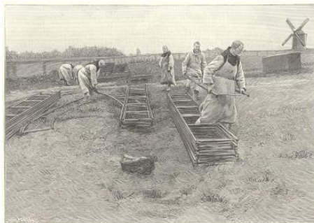
Trappists lay portable track
