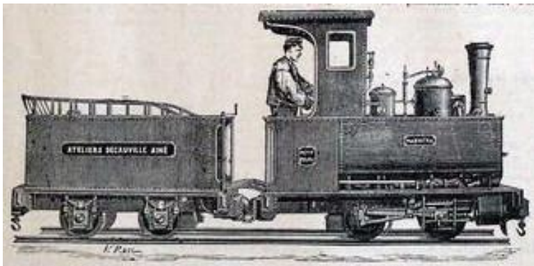
Oil-fired Decauville steam locomotive in Turkestan
