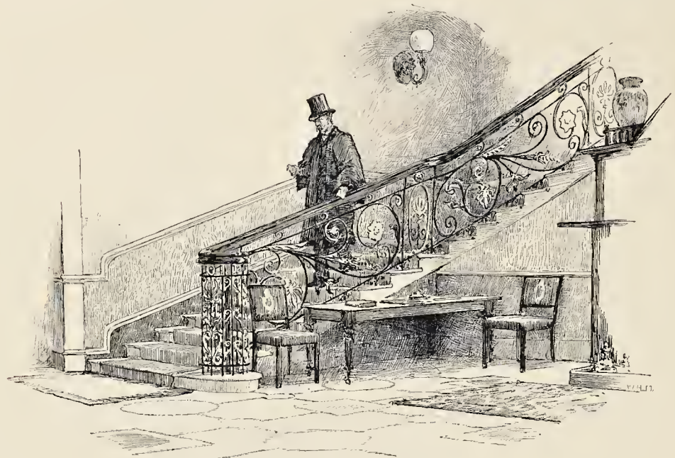
Principal Staircase, Birmingham Conservative Club.
