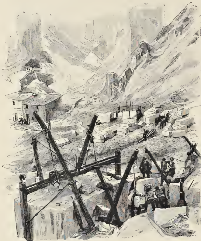
Fig. 1.—Sawing the Marble Blocks.
