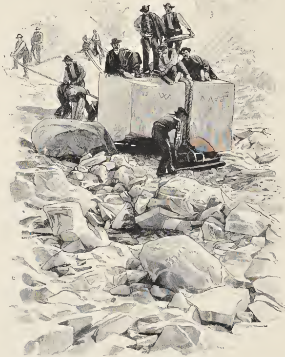
Fig. 6.—Transport of Marble Blocks by means of Ropes ("Lizza").
