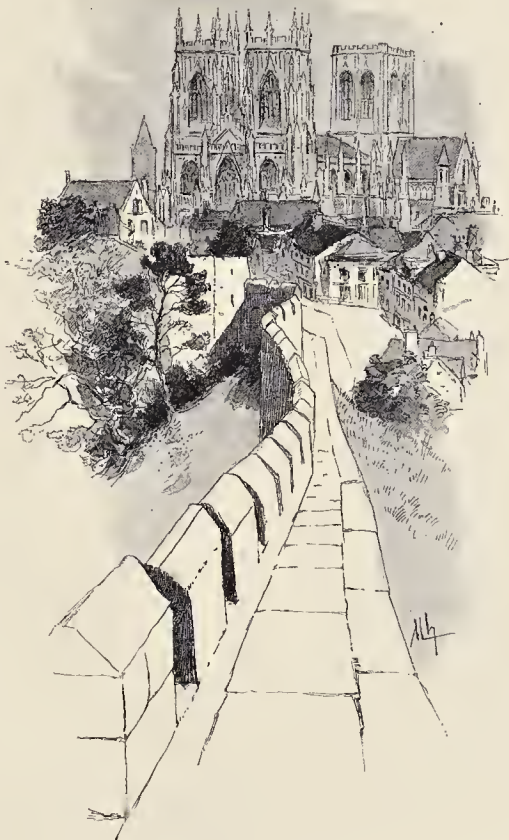
York Minster from the Walls.
