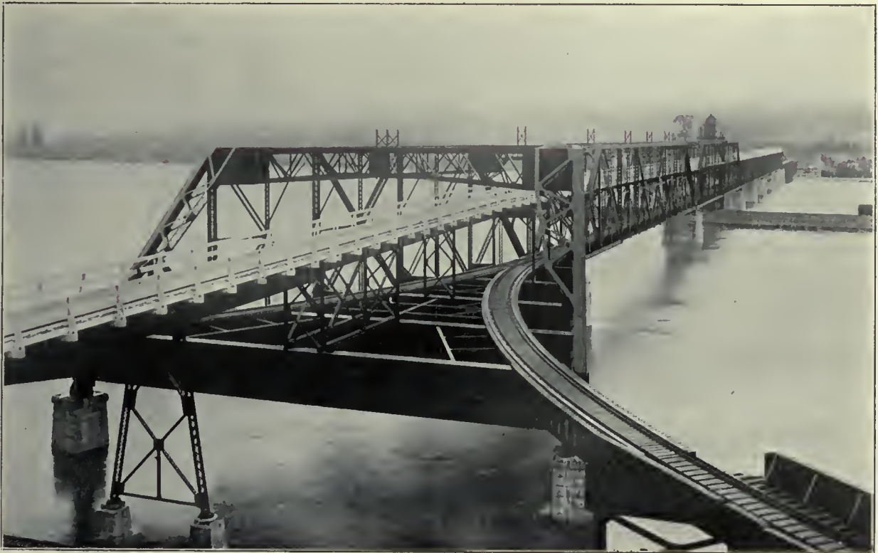
Combined Railway and Highway Bridge over the Fraser River at New Westminster, British Columbia, Built by Dominion Bridge Company, Limited, for the Government of British Columbia, 1905.
