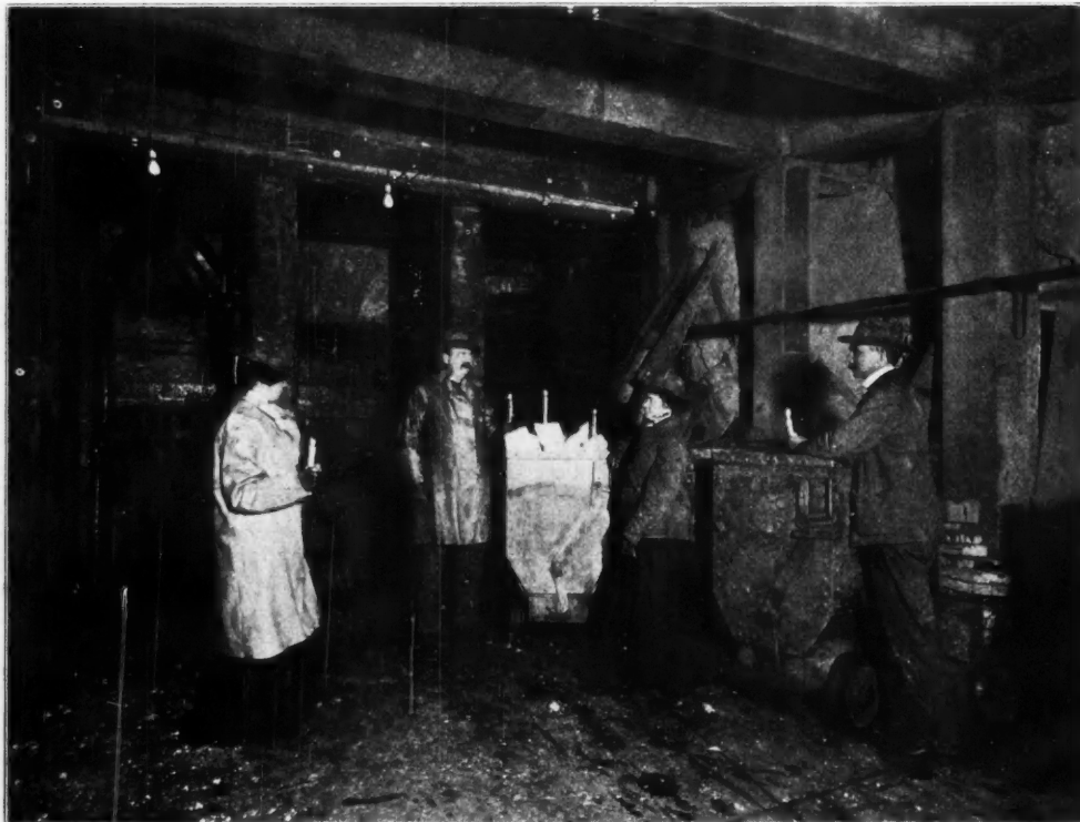
1,400 STATION, SPECULATOR MINE, BUTTE, MONTANA.
