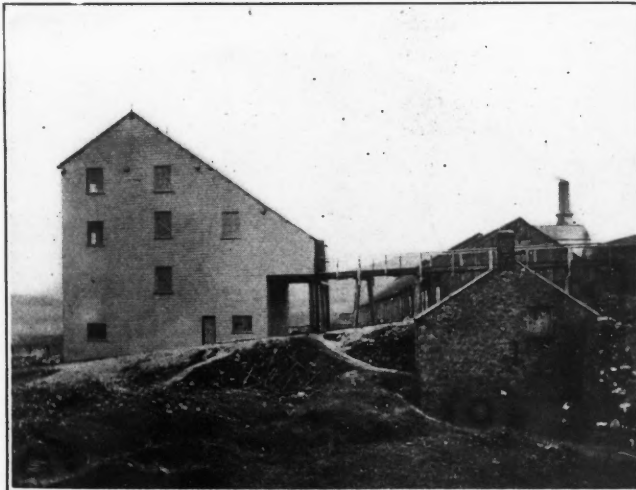
CONCENTRATOR HOUSE, DOLCOATH
