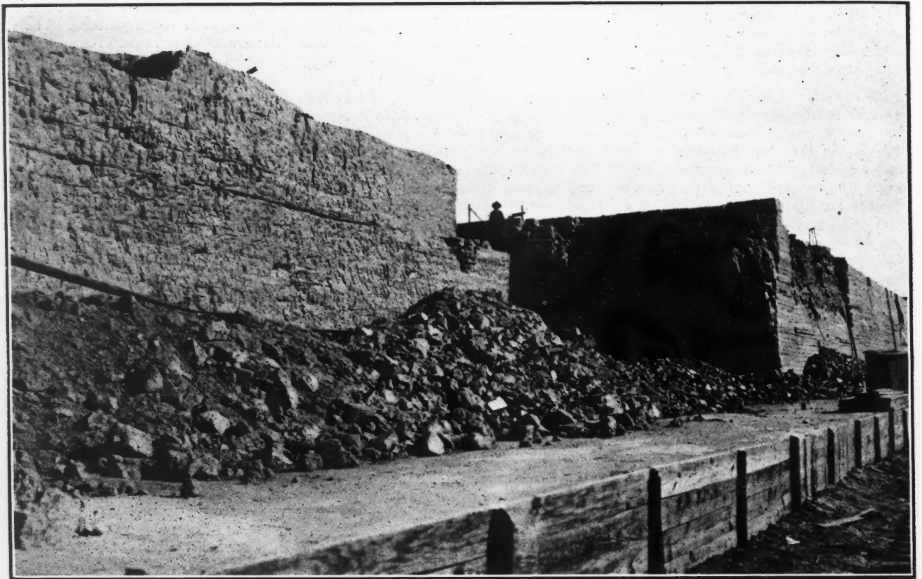
SULPHUR BIN STRIPPED OF ITS COVERING AFTER THE SULPHUR HAS SOLIDIFIED
