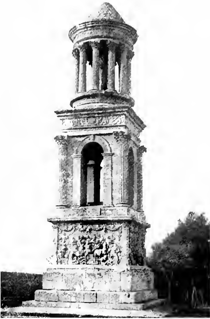
253—Monument of the Julii, Saint-Remy (Bouches-du-Rhône). (From photo.)
