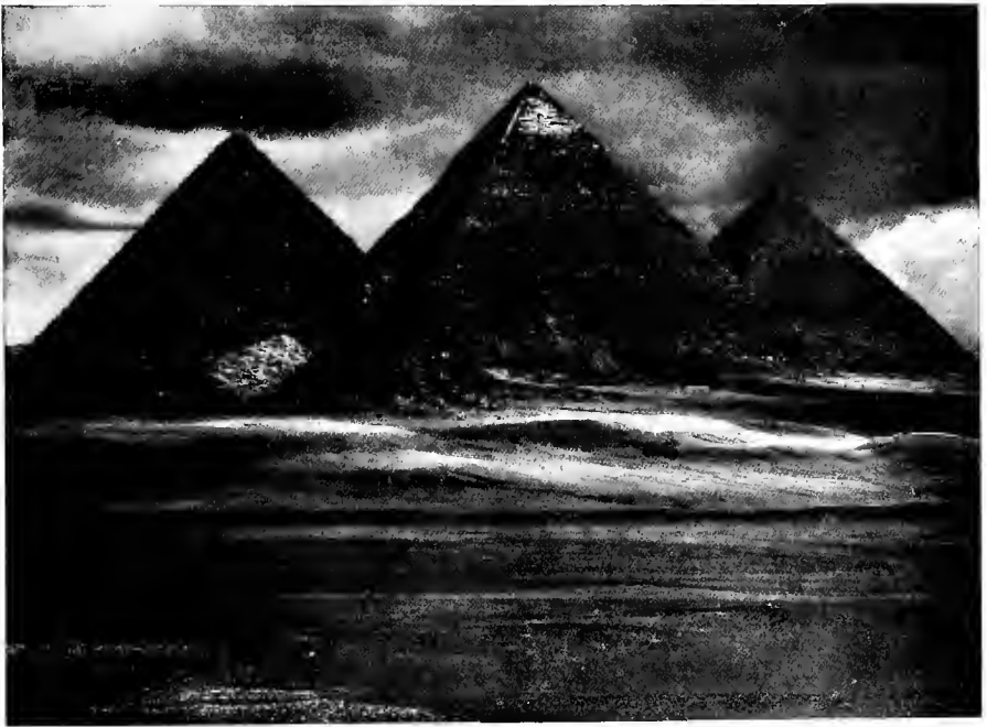
6—Stone Pyramids at Ghizeh. That of Khufu at the right, of Khafré in the centre and of Menkaure at the left: all of the Fourth Dynasty. The present heights are about 450, 445, 208 feet, from 10 to 30 feet being lost with the casing. Two small pyramids in front. (From photo.)
