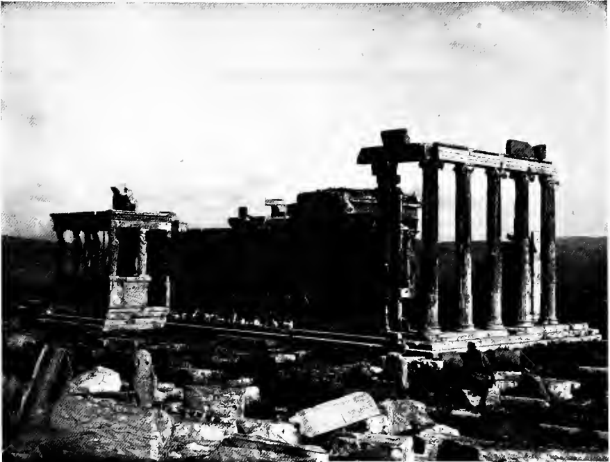
157—Erechtheion from south-east, showing hexastyle portico and Portico of the Maidens. (From photo.)
