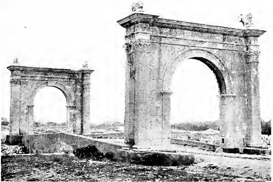
230—Flavian Bridge and Memorial Arches at Saint-Chamas. (Bouches-du-Rhône.) (From photo.)
