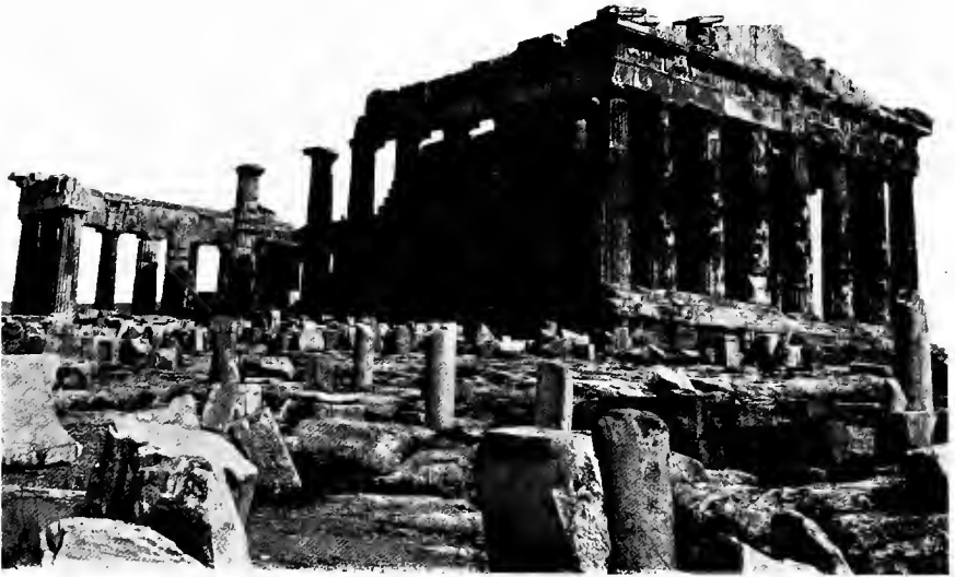
130—Parthenon from northwest. (From photo.)
