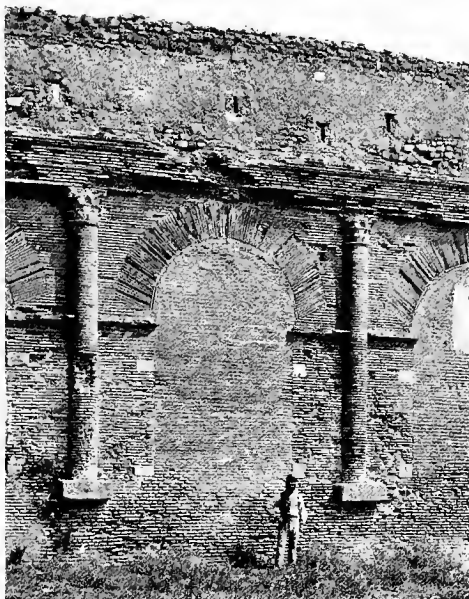
285—Amphitheatrum Castrense, Rome. Exterior brick facing. (From photo.)
