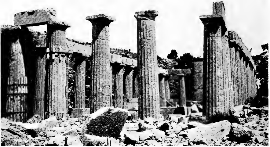
139—Temple at Bassai, from the south-east. (From photo.)
