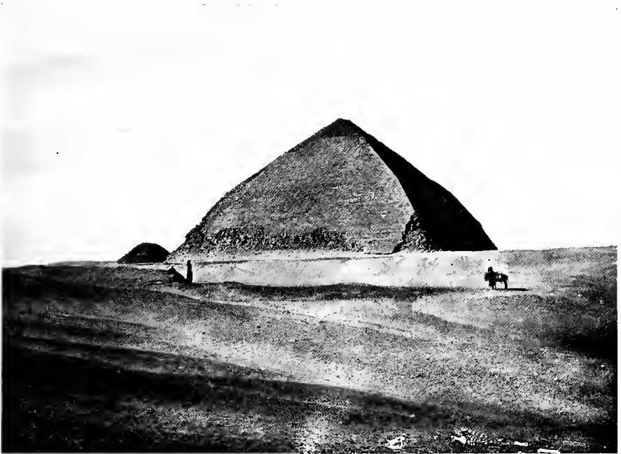
7—Stone Pyramid at Dahshur. With double slope. About 620 feet square and 320 feet high. (From photo.)
