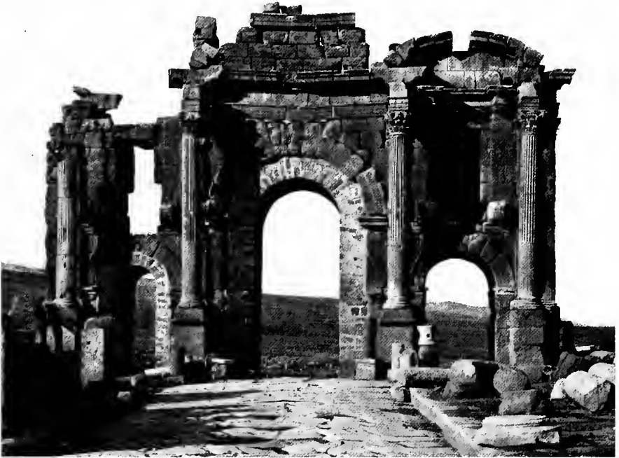
243—Arch of Trajan at Timgad, Algeria. (From photo.)
