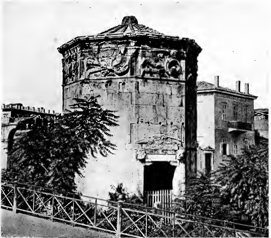
184—Building for water-clock, called Tower of the Winds, at Athens: The frieze bears symbolic figures representing the different winds, and the roof once carried a weather-vane. Height, including basement, 42 feet; diameter, 26 feet. (From photo.)
