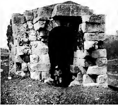
219—Ruined superstructure of tomb, ruins of Apamea, Syria. (From photo.)
