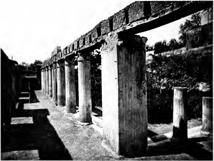
316—Peristyle of house in Herculaneum, called House of Argus. (From photo.)
