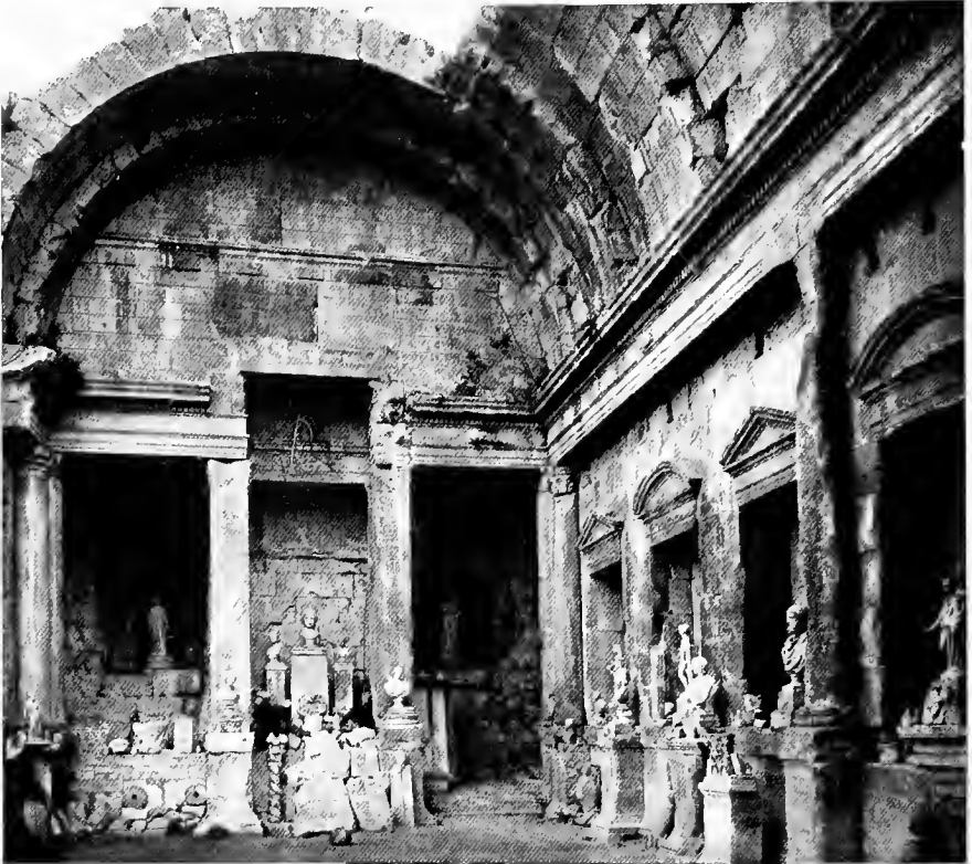
213—Building called Temple of Diana, or Temple of the Nymphs, Nîmes (Gard). (From photo.)
