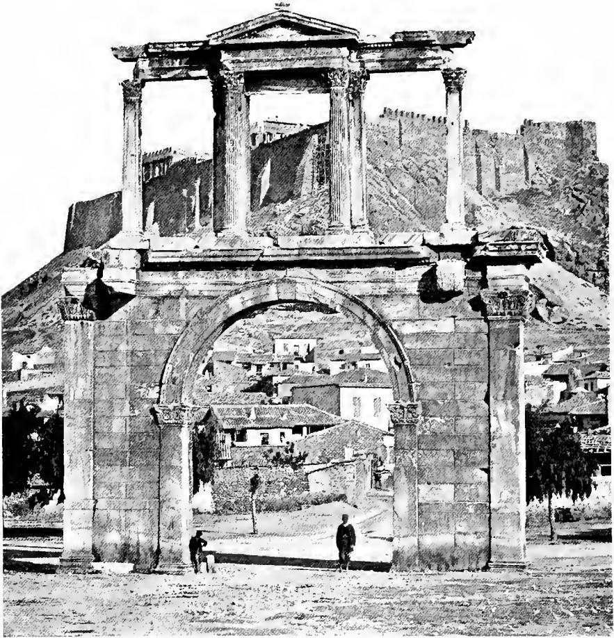
232—Roman gateway at Athens, called Arch of Hadrian. Looking northwest, from the site of the later Roman city and toward the Greek city and the Acropolis. The building seen through the middle opening of the upper story is the Parthenon. (From photo.)
