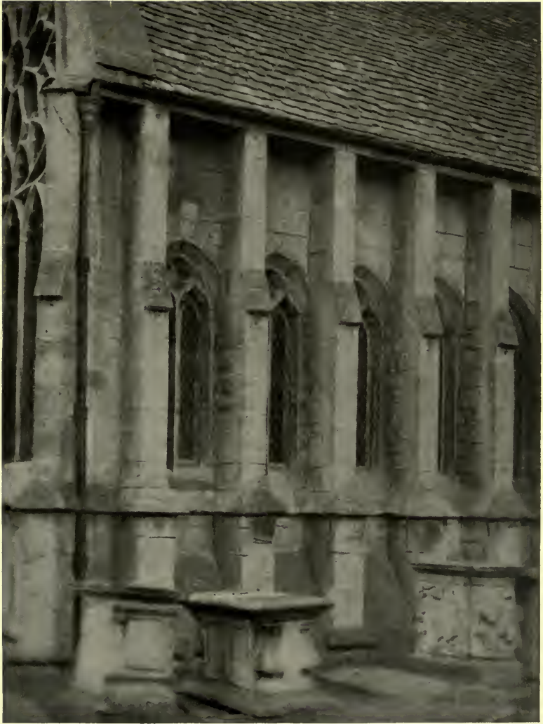
MINCHINHAMPTON CHURCH, SOUTH TRANSEPT. Exterior
