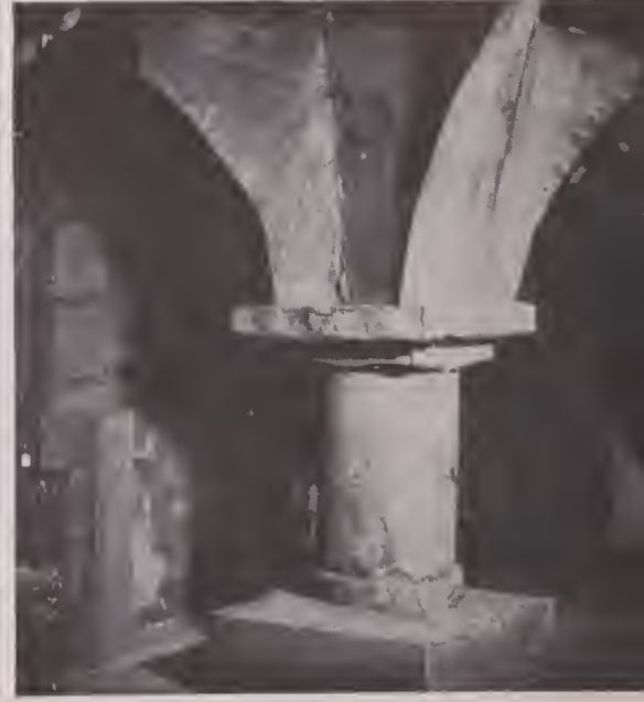
MASONRY detail also constructed in "garage" studio by Gospel Film's ingenious craftsmen, again using wallboard paste, paint and plaster.
