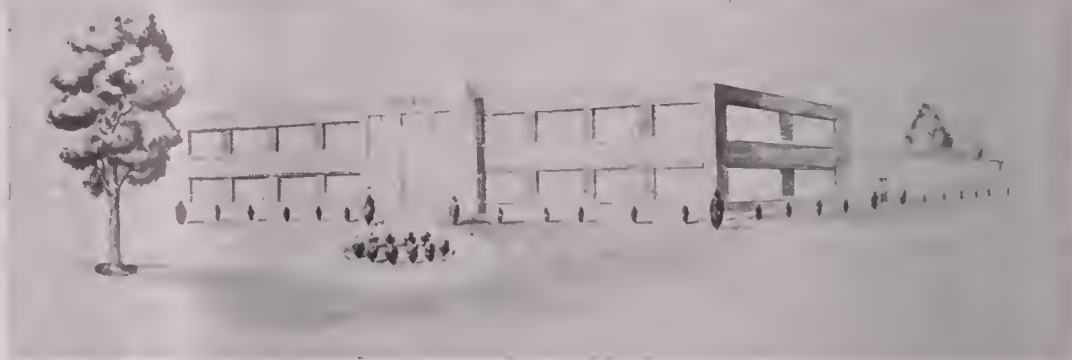
The new, modern Goerz plant in Inwood, Long Island, N. Y.
