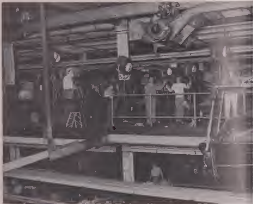
LOCATION INTERIORS in large factories present the greatest problem for the industrial film cameraman. A wide array of lighting units are necessary to cover the vast areas and to spread sufficient
