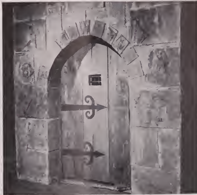
. . . of door, and change of camera angle and lighting for still another sequence. "Stone" is wallboard panels cemented to flats and painted.
