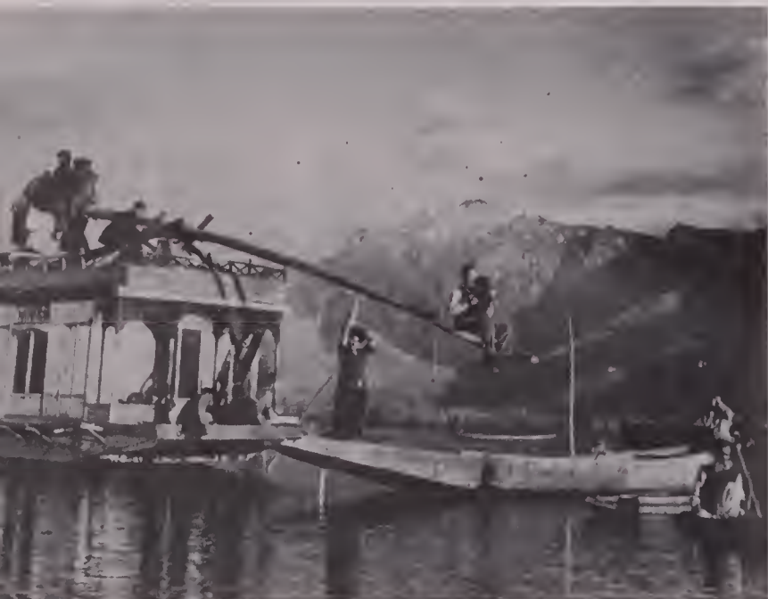
A NOVEL camera boom was made from a telegraph pole. Cameraman Marconi sits precariously on the far end to make a vital crane shot, while group of assistants lend balance at the other end.
