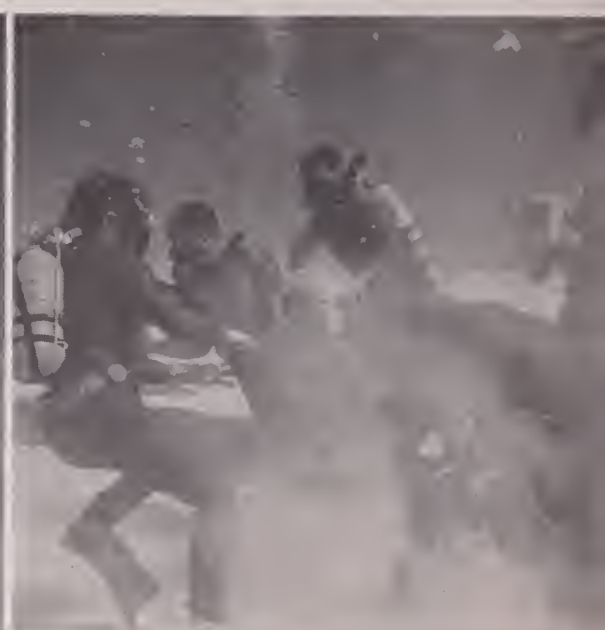
6 Heavy hemp mat is placed on ocean floor to reduce amount of sand kicked up by divers, thus increasing production time underwater.
