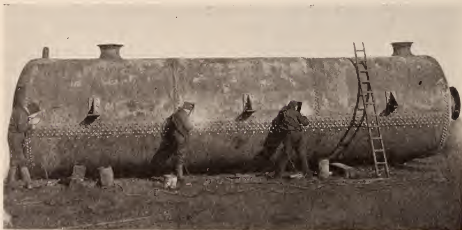
Figure 4—Welding seams in large oil tank
