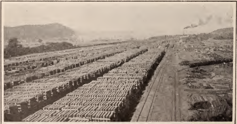
Seasoning Ties at the Timber Preservation Plant, Green Spring, W. Va.
