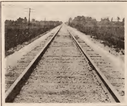
Standard track recently completed west of overhead bridge at Lyndon, Ohio
