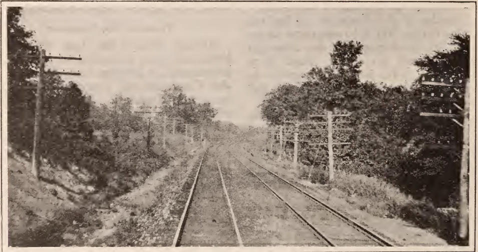
Wherever the steel rails lead, there follow the long lines of wires which make possible their safe and efficient operation
