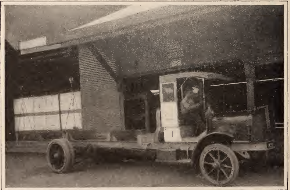
Showing motor truck chassis leaving for adjacent superstructure to receive another unit demountable body
