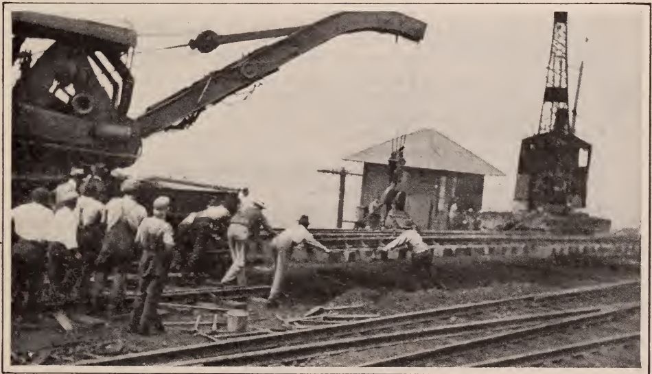
New Method of Installing Switches
