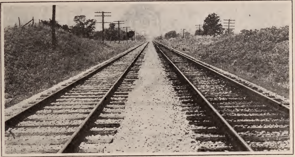
Looking west on eastbound, from west of west switch, Pataskala, Ohio
