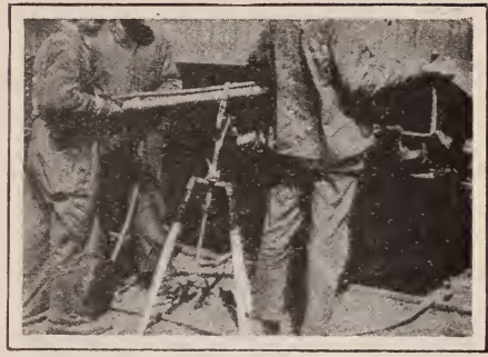
No. 8—Tool Support Stand with Rivet Buster
