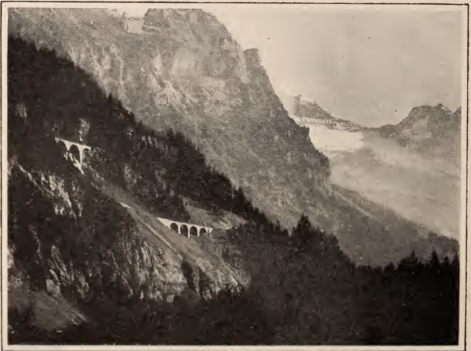
The Loetschberg Railway in the Kandersteg Valley, Switzerland, where it is seen passing on viaducts at different altitudes
