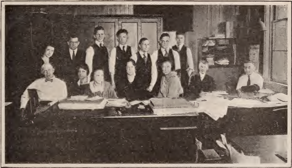
Office Force at Massillon Freight House
