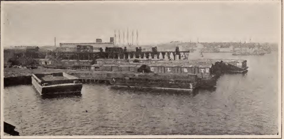
Site secured for the American Sugar Refining Company Plant at Locust Point, Baltimore
