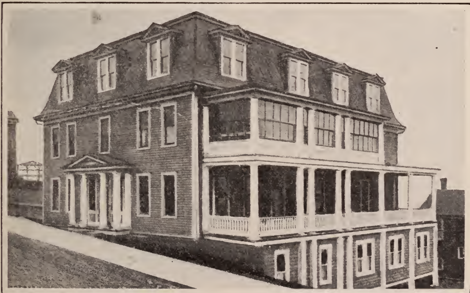
The Hoffman Hospital in Keyser (See Keyser Notes)
