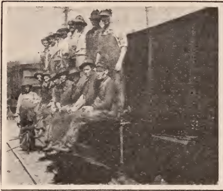
No. 2—The scaffold is strong enough to support ten men, an oil tank, stand and burner
