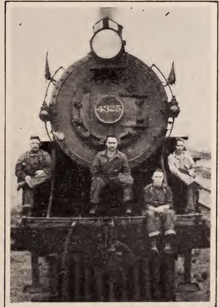
Akron Holloway Crew
