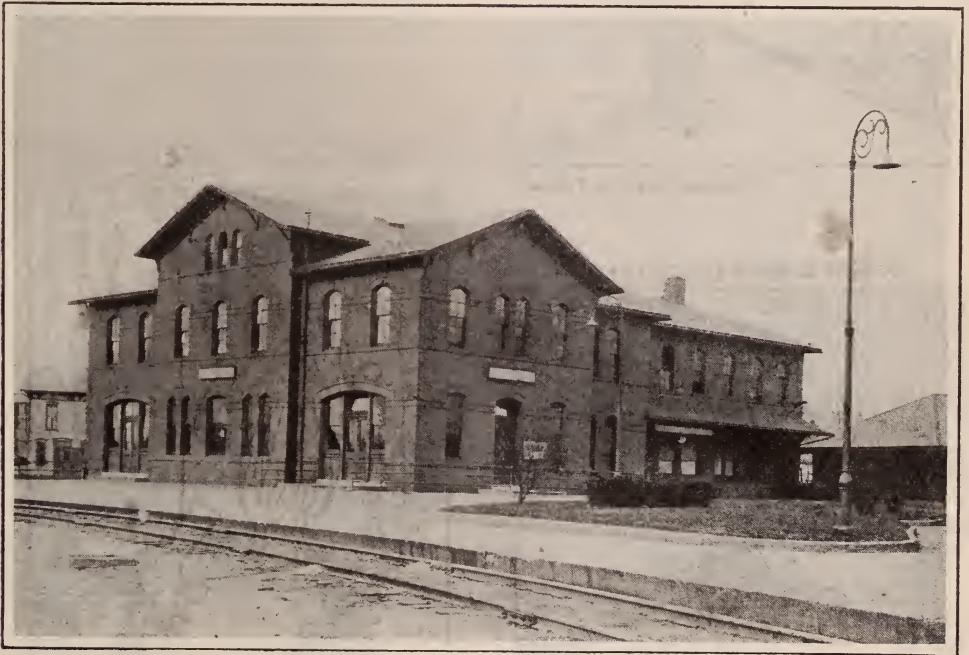
PASSENGER STATION AT NEWARK, OHIO—NEWARK DIVISION
