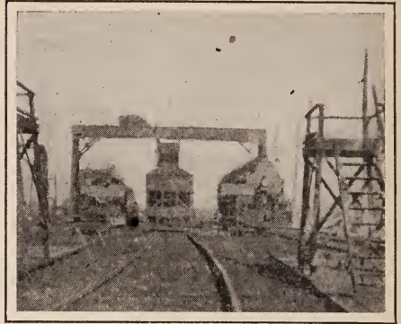
New Ash Hoist at Keyser
