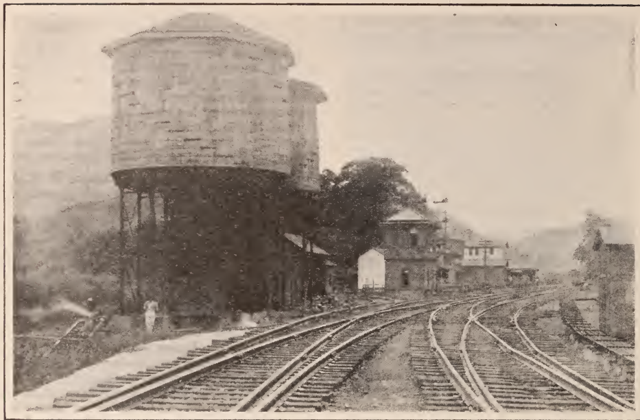
Main Track approaching Glover Gap Station and "GO" Tower, Wheeling Division
