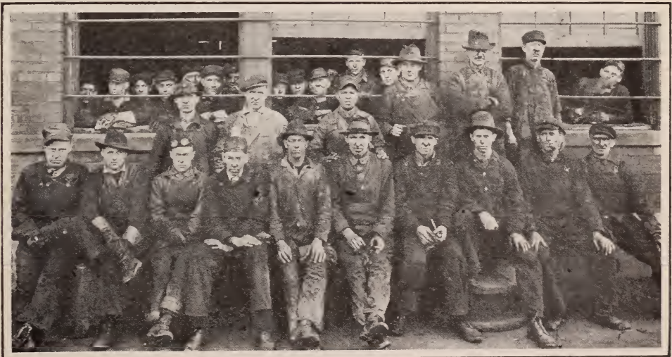
Boiler Gang at Benwood Shops
