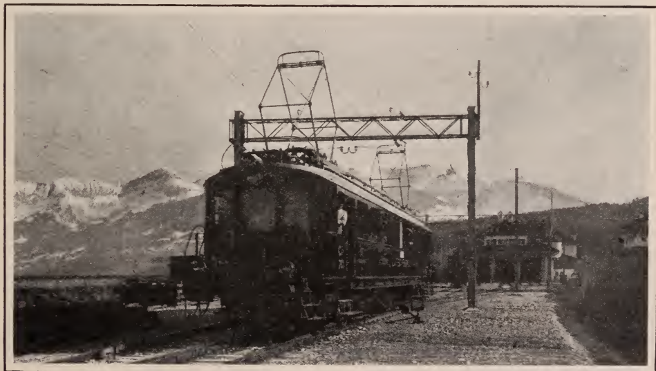
2,000 horsepower electric locomotive on the Loetschberg Line, Switzerland
