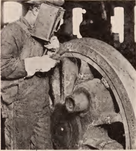
Figure 8—Repair to driving-wheel spokes
