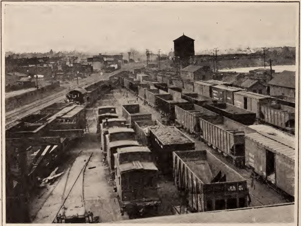
General View from Yard Office
