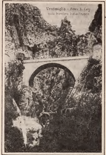
The Bridge Connecting France and Italy at Ventimiglia
