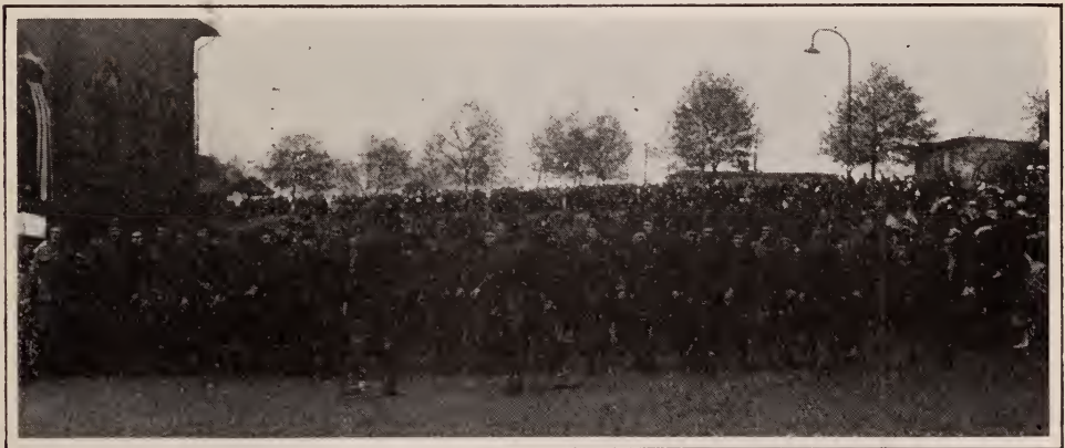
• HOME"—After eighteen months in the trenches
