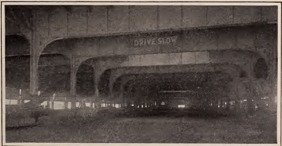
Interior of pier—first deck, looking east
