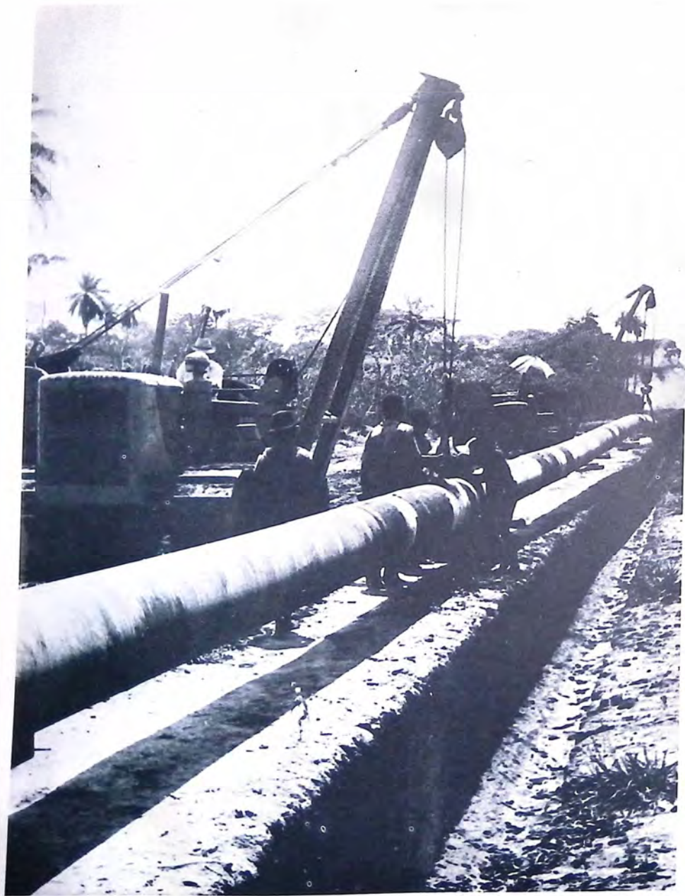
Laying oil pipelines
