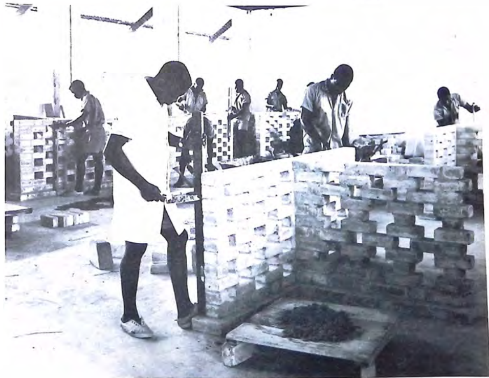
A bricklaying class at the Government Trade Centre, Sapele
