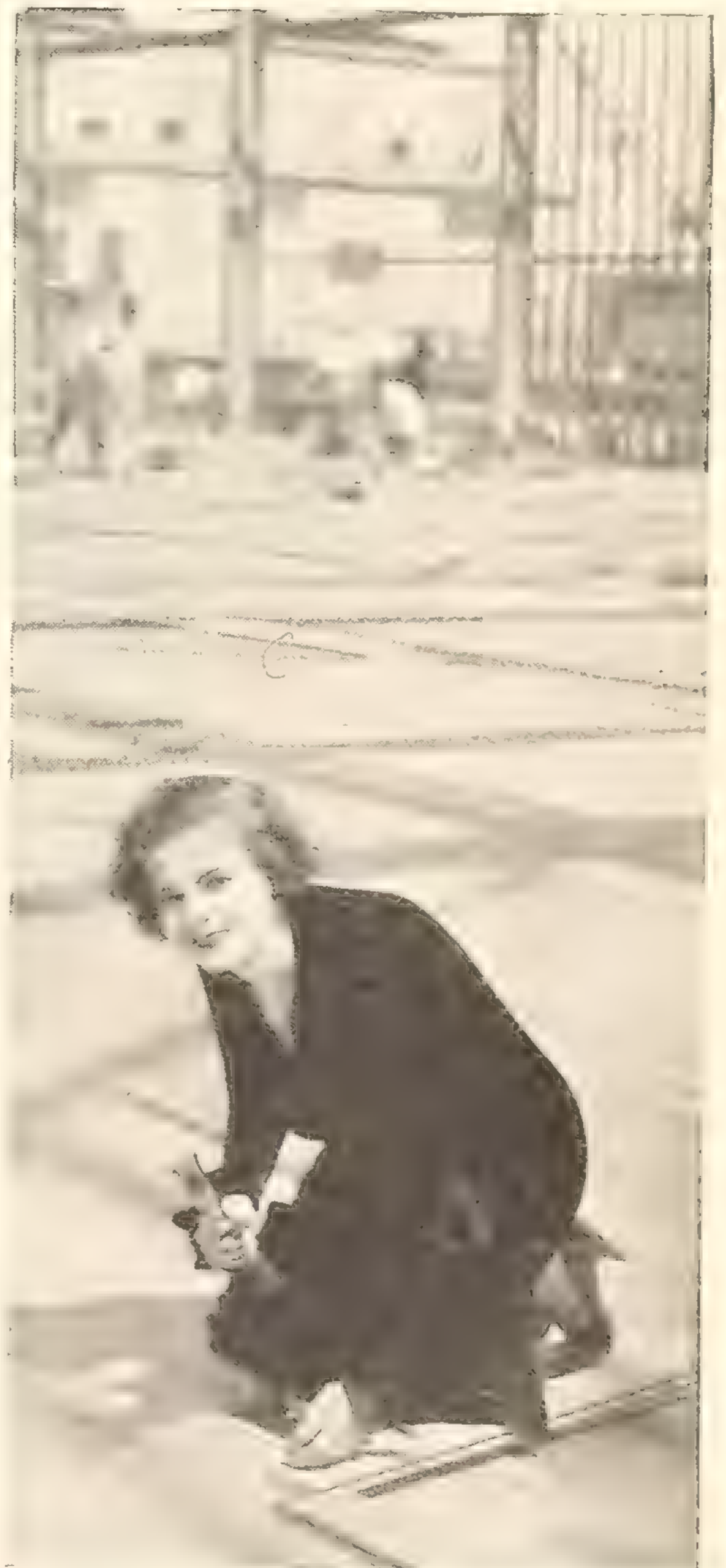
“Vera Reynolds finishes the largest covered stage in the world, over an acre.
