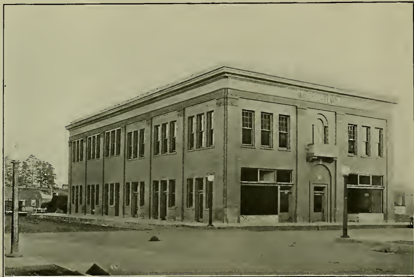
A Most Creditable Edifice
