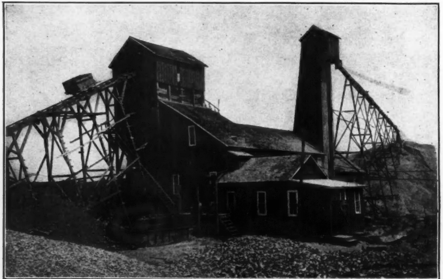
NO. 2 MILL AT THE MOLER-SMITH MINE, JOPLIN, MO.
