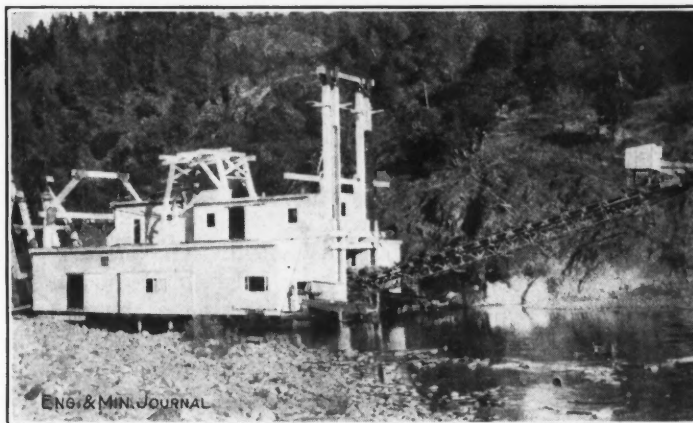
PACIFIC NO. 1 DREDGE OPERATING ON AMERICAN RIVER, CALIF.
