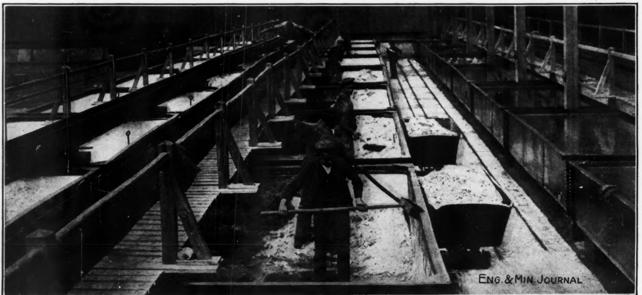
DIGGING OUT THE CRYSTALLIZED POTASSIUM SALTS AT A GERMAN POTASH WORKS Copyright by International News Co.
