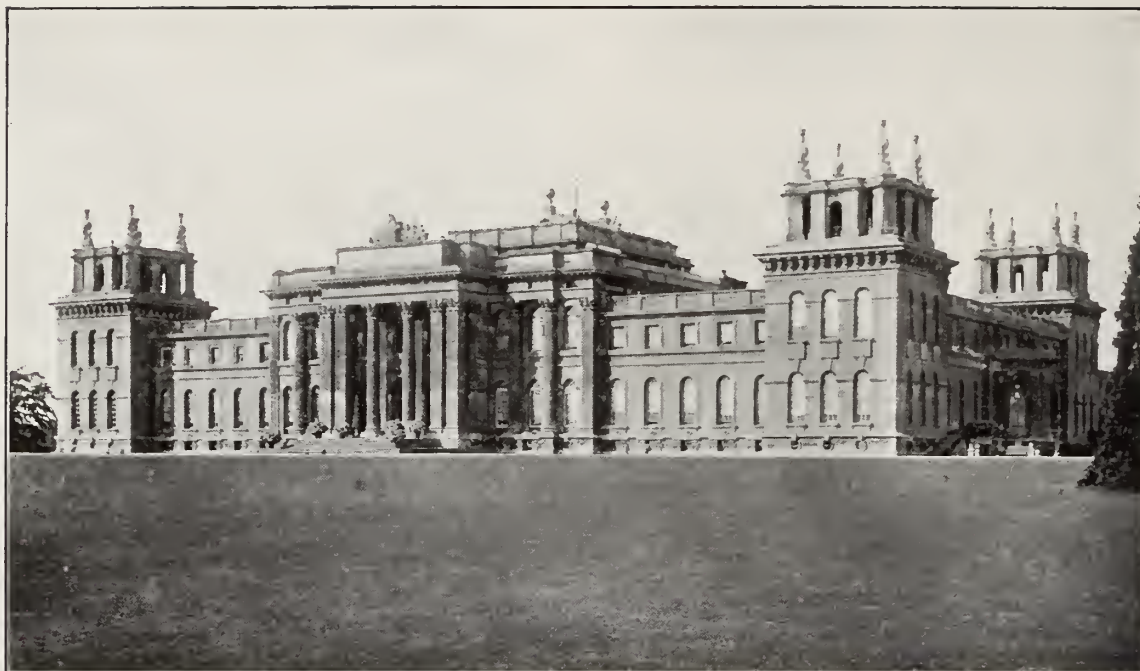
Blenheim Palace. The South Front.
