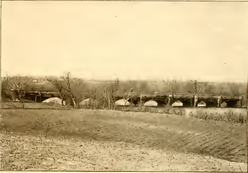
FIG. 1.—MONOCACY AQUEDUCT, WHITE QUARTZITE FROM BELT'S QUARRY.
