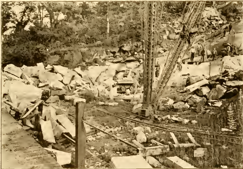
FIG. 2.—SANDSTONE QUARRY, POINT OF ROCKS, FREDERICK COUNTY.
