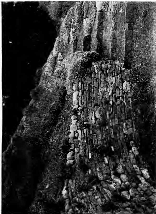
FIG. 17.—A DRY WALL SHORTLY AFTER CONSTRUCTION.
