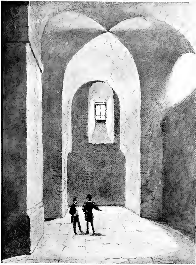
17. VAULTED ROOM IN THE CRYPT OF THE WHITE TOWER, IN WHICH THE RACK STOOD. From a drawing in the Gardner Collection.
