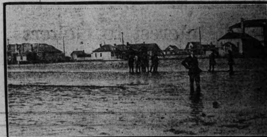
Brooklands, Manitoba, is one of the many districts of that Province which are under water as a result of Spring floods. Many Brookland homes present the appearance of islands in a large lake.
