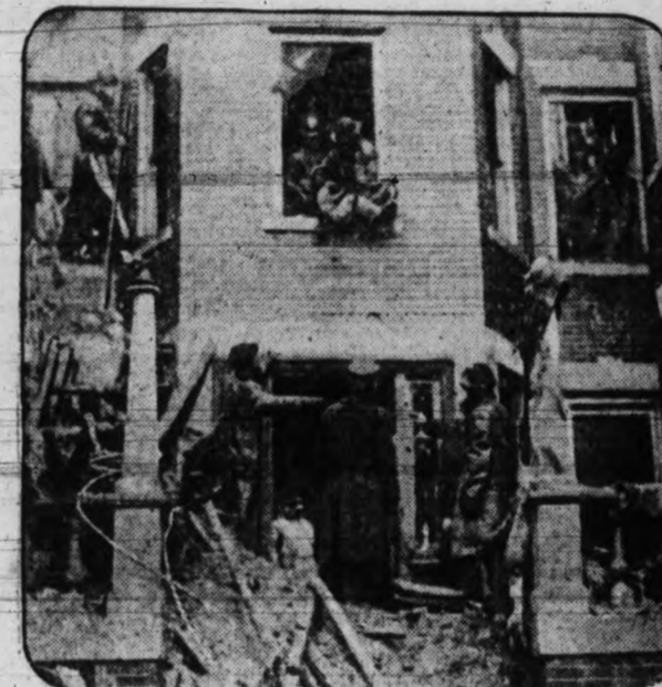
Firemen and police removing one of the five victims of a fire that swept an apartment house at Lynn, Mass. There were no fire escapes and the flames swept so rapidly that the tenants were trapped.
