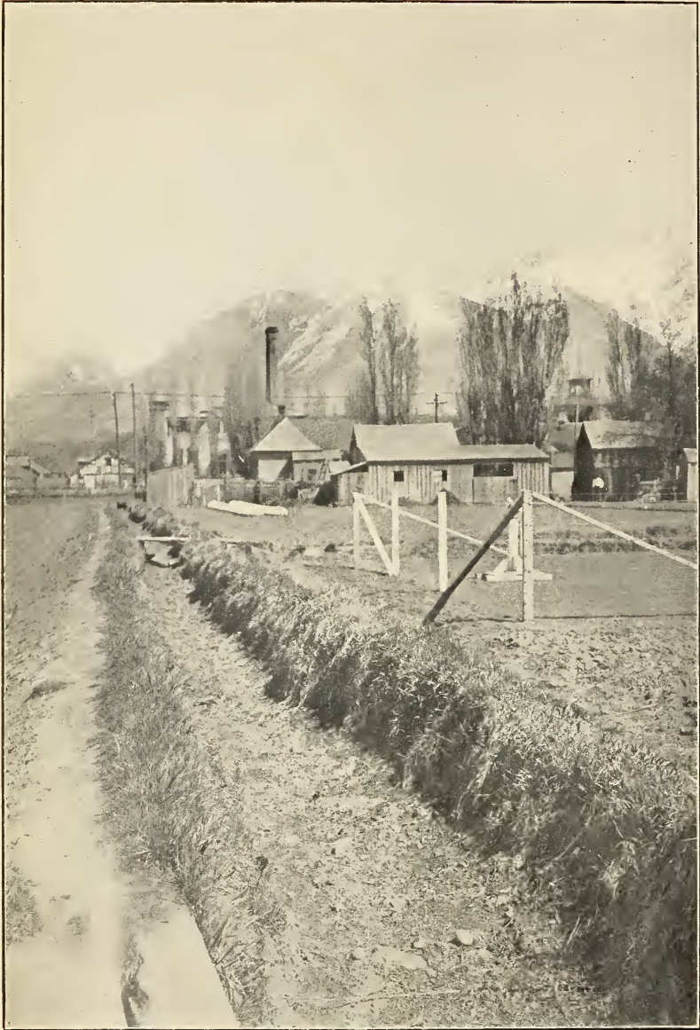
PERMANENT LATERAL IRRIGATION DITCH WHOSE BANKS ARE KNIT TOGETHER WITH GRASS; EASILY KEPT FREE FROM WEEDS.
