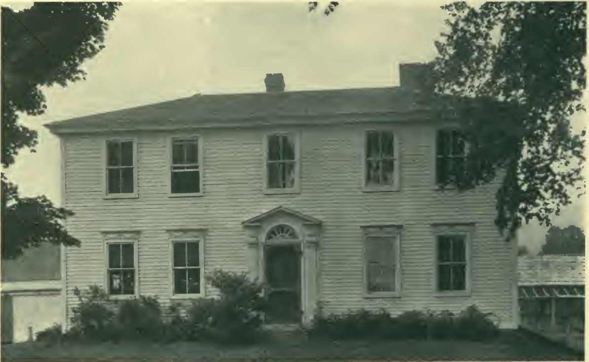
HOUSE AT WEATHERSFIELD, VERMONT.
