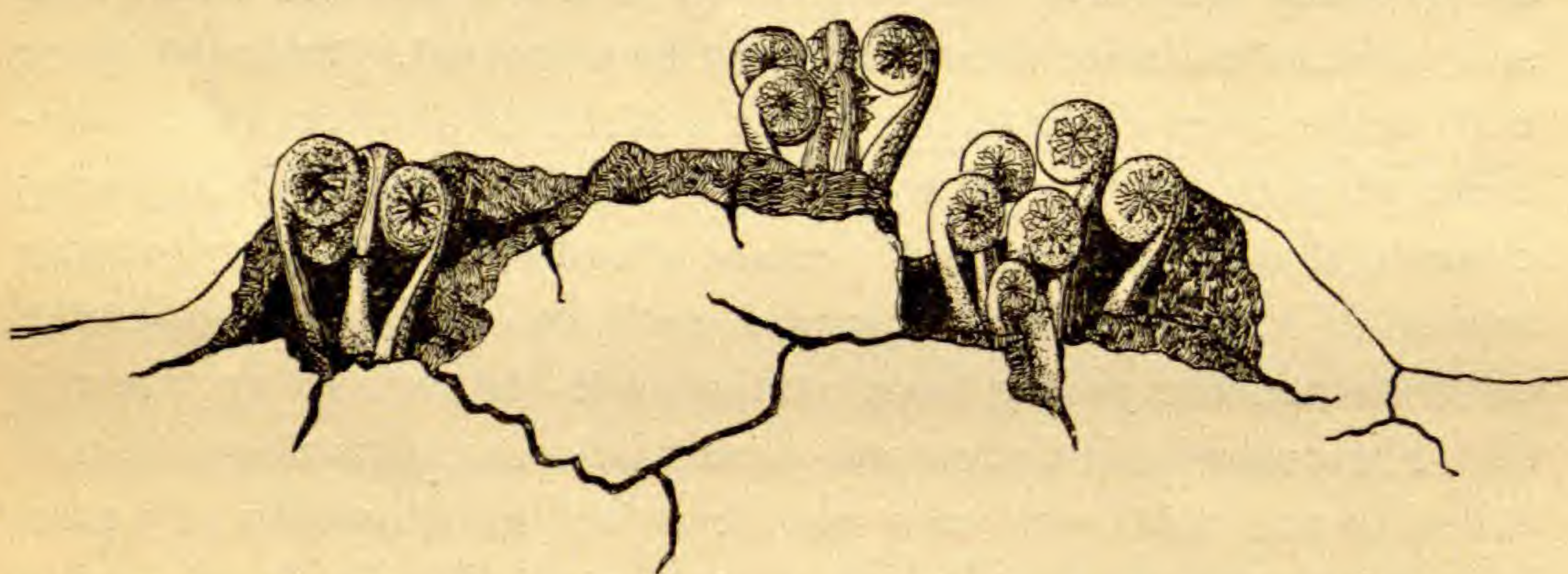
FIGURE I. The rupturing of concrete by the young fronds of ostrich ferns ( Onoclea Struthiopteris Hoffm.).
