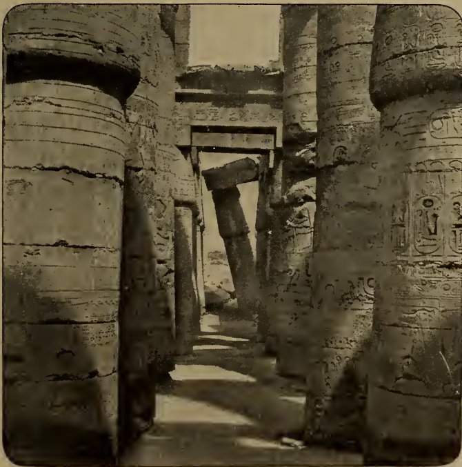
THE LEANING COLUMN.
