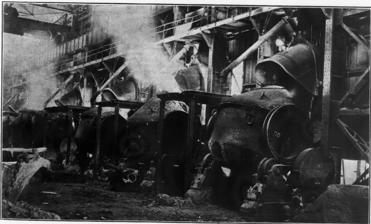
CONVERTERS AT THE CALUMET & ARIZONA SMELTER, DOUGLAS, ARIZ.
