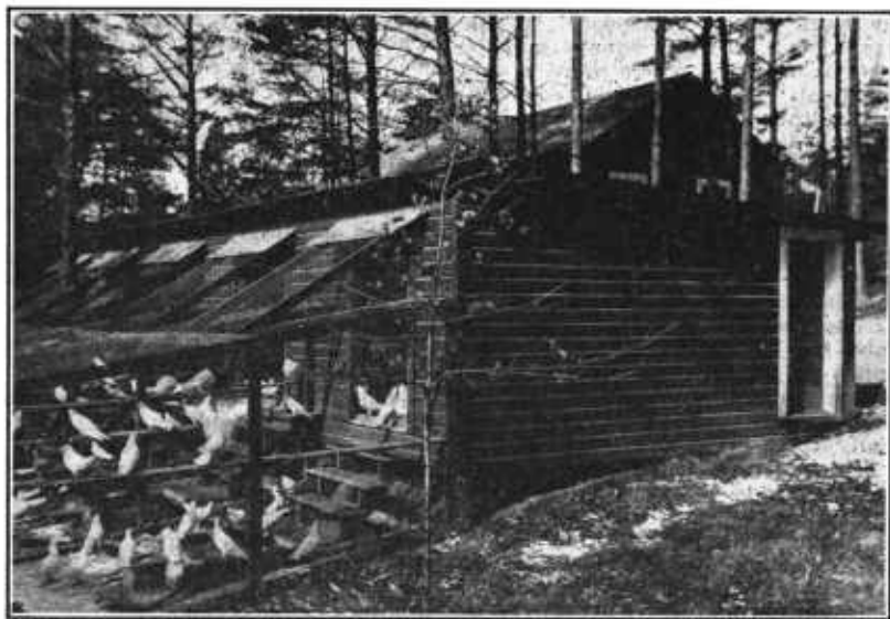
FIG. 8.—Shed-roof pigeon house with partly open front. Attached fly contains a concrete bathing and drinking basin supplied with running water
