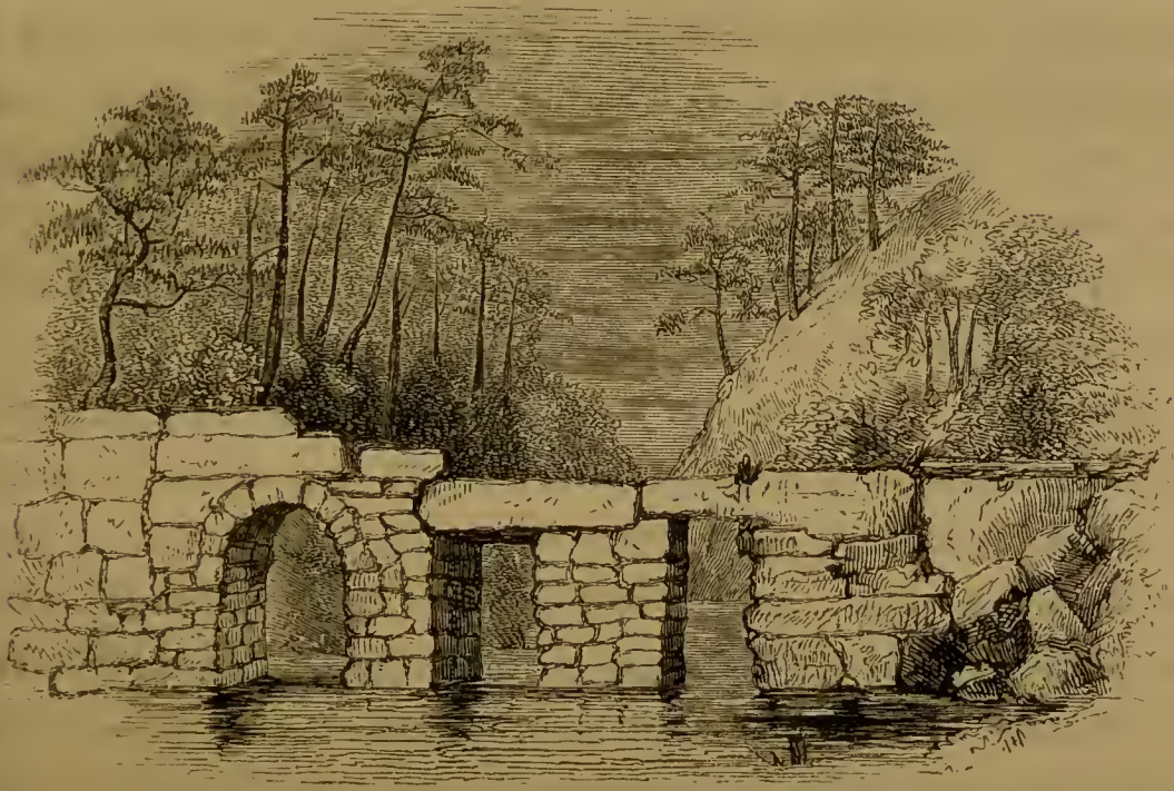
OLD BRIDGE AT AMWEE.
