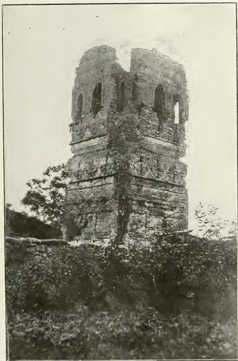
DRUM TOWER, T'AI P'ING KUNG Photo by Banzi & Co. Kuling.
