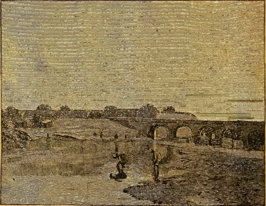
THE RAILROAD BRIDGE OVER THE JUMNA AT DELHI.
