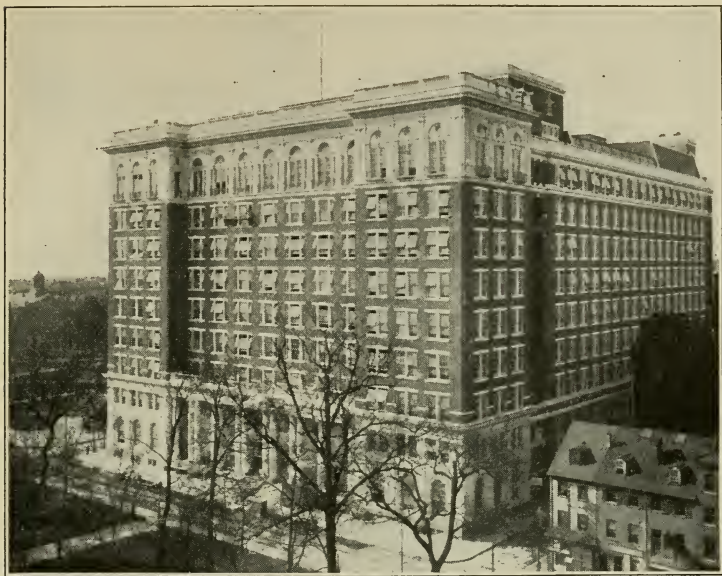
Curtis Publishing Company Building S. 6th, S. 7th and Walnut Streets
