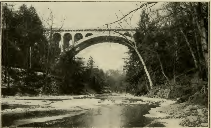
Walnut Lane Bridge across the Wissahickon
