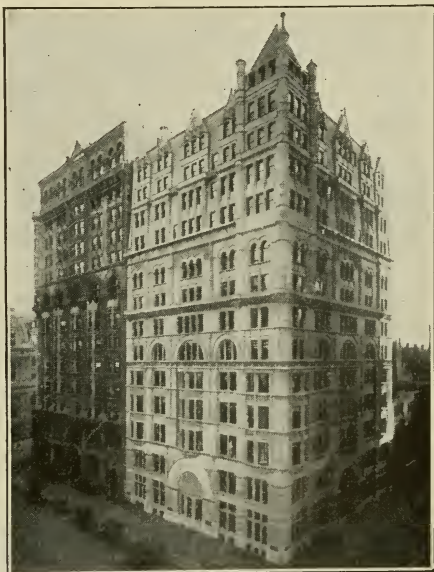
Franklin National Bank Building Betz Building on the Left S. Broad and Chestnut Streets Page 39
