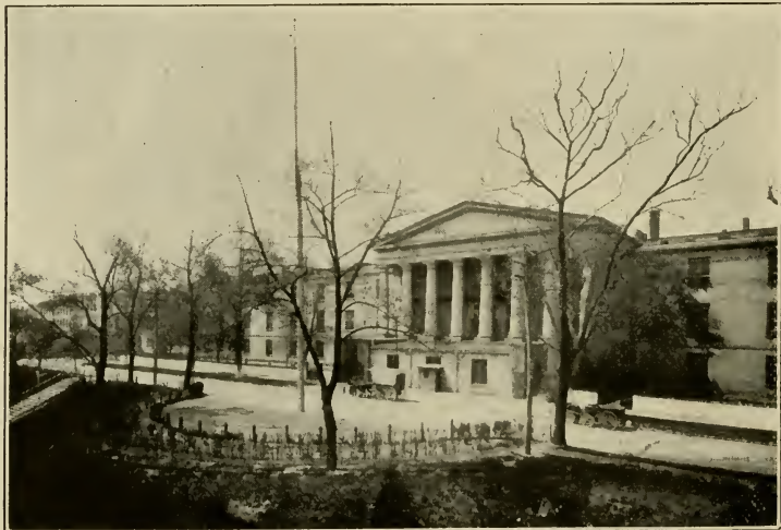
Philadelphia General Hospital and Almshouse S. 34th and Pine Streets
