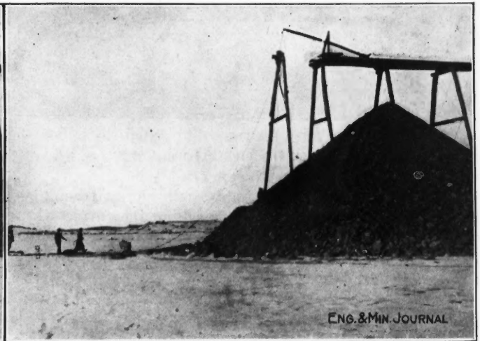
THE BENT IN PLACE
