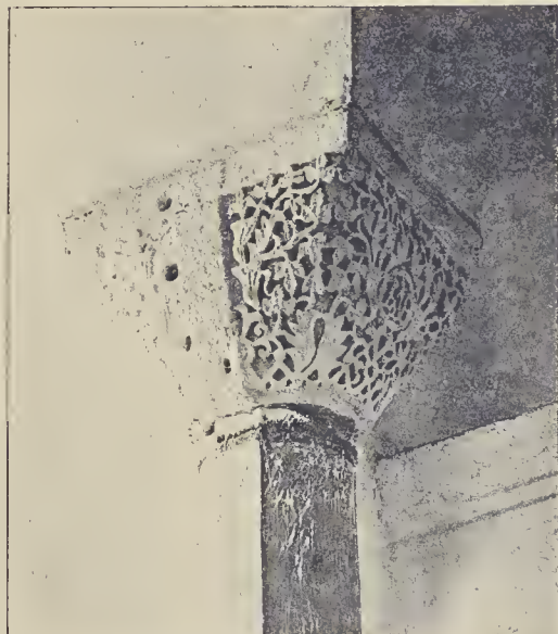
CAPITAL TO RECESS IN SOUTH AISLE.
