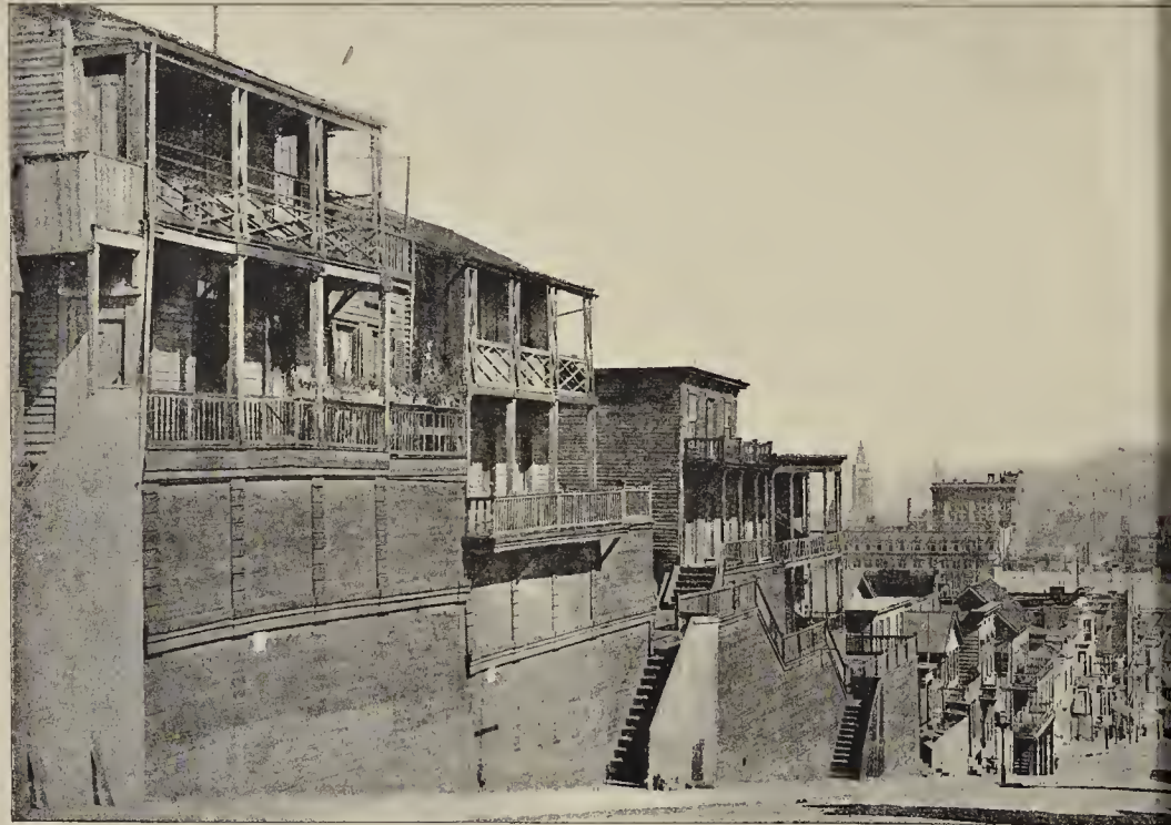
Tottering Wooden Shanties on the Nob Hill Grade, forming the Fuse which led the Fire up to the Mansions on the Summit.
