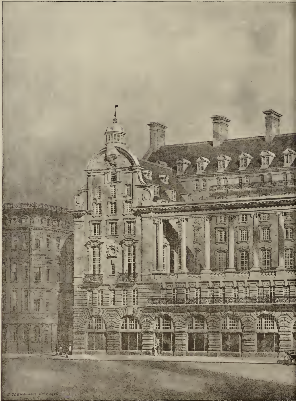
FRONT OF THE PICCADILLY HOTEL—NOW BUILDING FROM FROM DESIGNS PREPARED FOR THE OFFICE
