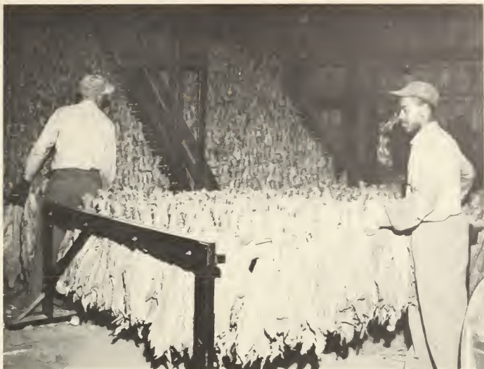
Figure 36.--Unstemmed burley tobacco entering a redrying machine in a redrying plant.
