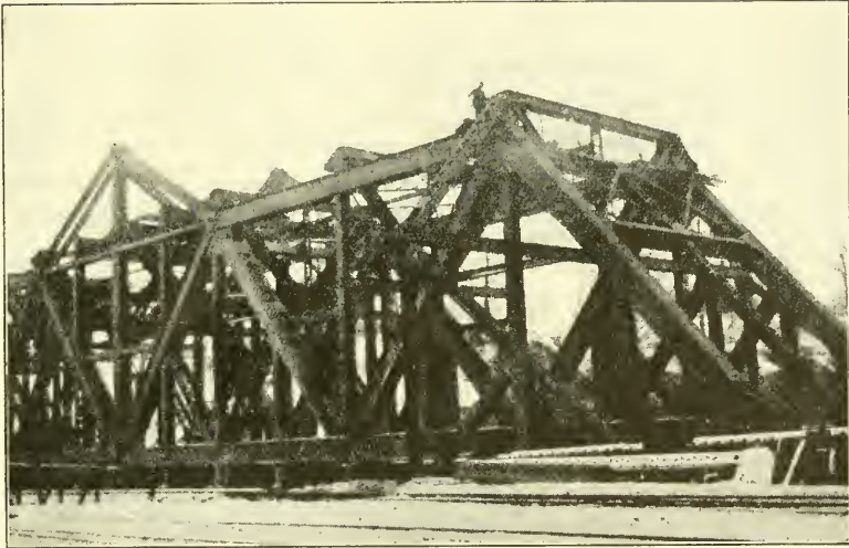
FIG. 5.—CONNEAUT DRAW SPAN DURING ERECTION. COMMENCING TO PLACE THE OVERHANG.
