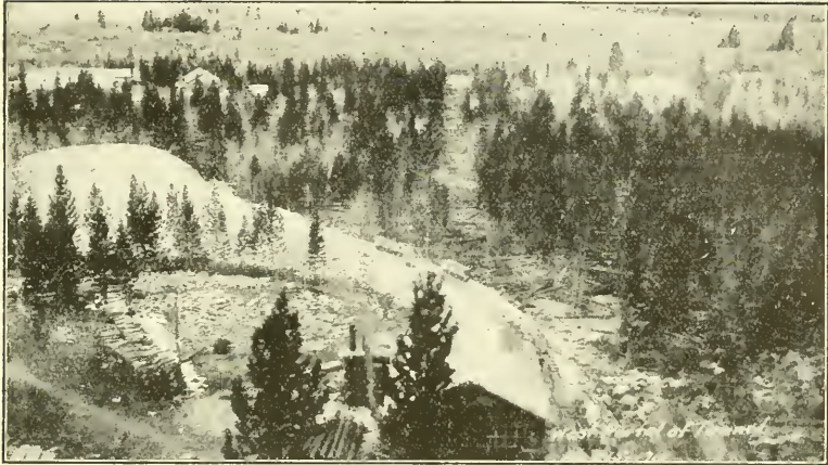
FIG. 7.—WEST PORTAL CAMP AND DUMP.
