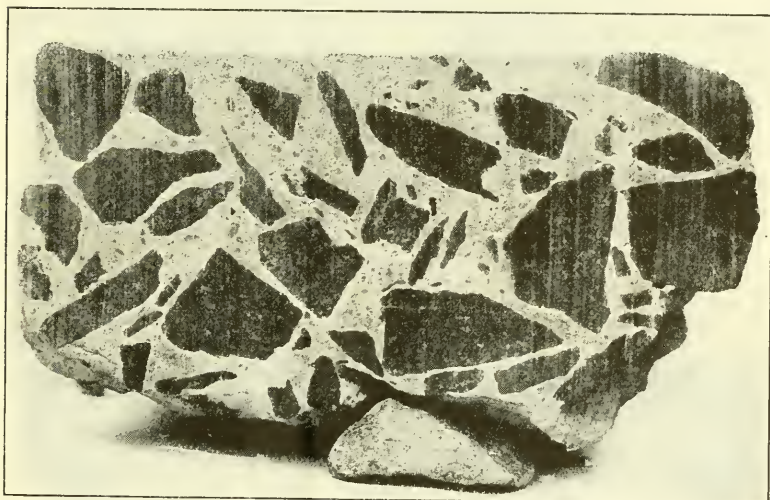
FIG. 25.—SEC. 13.—“HASSAM” CONCRETE PAVEMENT, BUILT BY FORCING INTO VOIDS OF STONE BY PRESSURE MACHINE, MORTAR OF 1\frac{3}{4} PARTS SAND TO 1 PART PORTLAND CEMENT.
