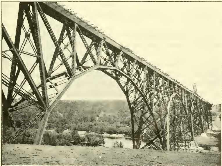
FIG. 6.—THE CLOSURE OF THE CENTER SPAN.
