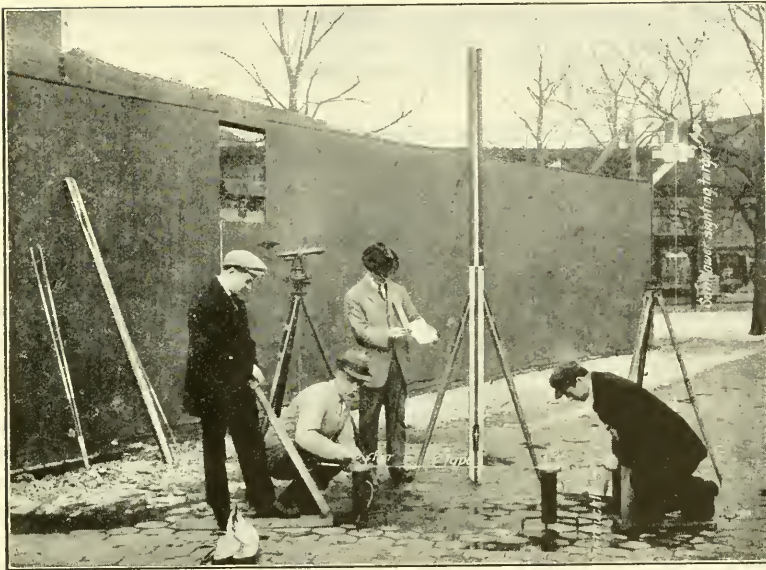
FIG. 14.—APPARATUS USED FOR BASE-LINE TAPING, FOR CITY TUNNEL, CATSKILL AQUEDUCT.
