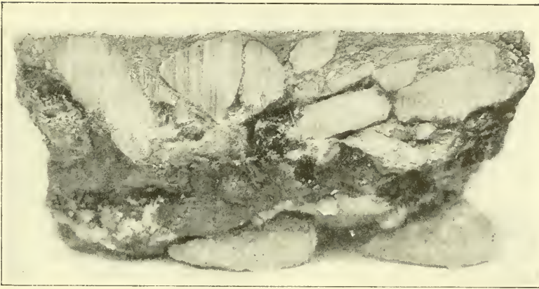
FIG. 27.—SEC. 16.—BITUMINOUS PAVEMENT, BUILT BY PENETRATION METHOD. 1½-IN. TRAP ROCK, ROLLED TO A DEPTH OF 3 IN., 1½ GAL. BERMUDEZ ROAD ASPHALT APPLIED, LAYER OF CHIPS ROLLED, ½ GAL. BERMUDEZ ASPHALT APPLIED, OVER WHICH A LAYER OF CHIPS WAS ROLLED
