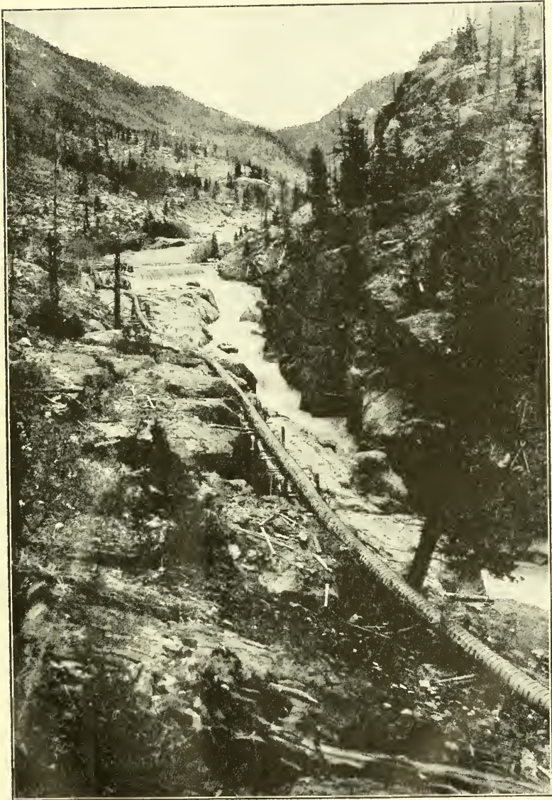
FIG. 6.—DAM AND PIPE LINE FOR POWER-PLANT ON POUUDRE RIVER, EAST PORTAL.
