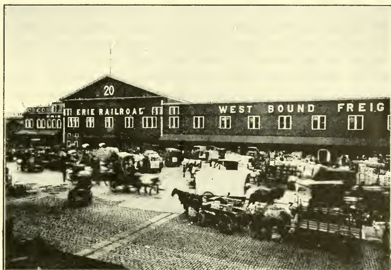
FIG. 4.—CONGESTION OF TRUCKS ON NORTH RIVER MARGINAL WAY.
