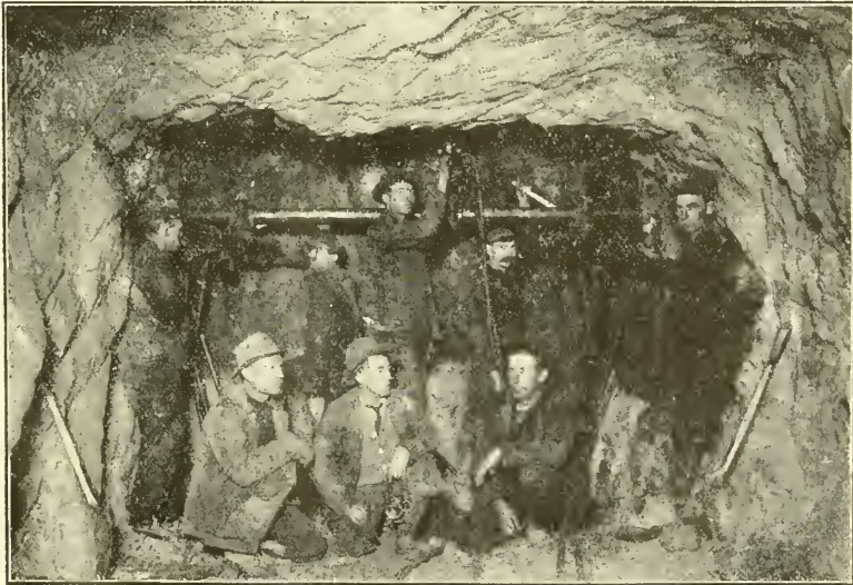
FIG. 8.—DRILLS ON BAR, AT EAST PORTAL HEADING.
