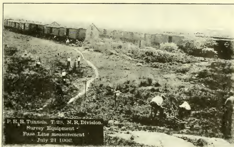
FIG. 10.—BASE LINE MEASUREMENT. PENNSYLVANIA RAILROAD TUNNELS.
