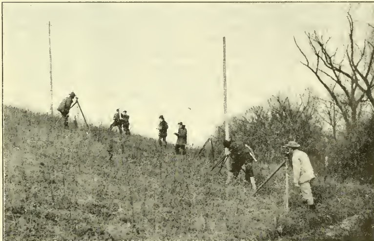
FIG. 15.—APPARATUS USED FOR BASE-LINE TAPING, RONDOUT PRESSURE TUNNEL.
