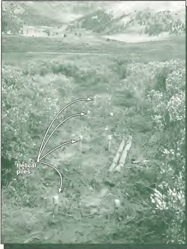
Figure 37—Helical piles installed in Colorado. The saddles are not yet attached. The ends are covered with temporary plastic caps for safety.
