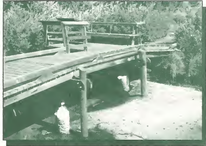
Figure 44—Know your soil conditions. Concrete end-bearing piles settled 1 to 2 feet here, and had to be replaced with these log friction piles.
