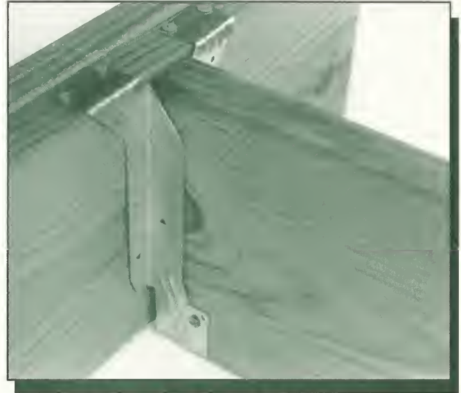
Figure 54—Supporting joists with truss hangers helps keep a boardwalk closer to the ground.
