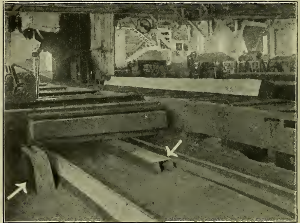
Fig. 12. Carriage Feed Cable Sheave and Set Works Sheave Guarded.
