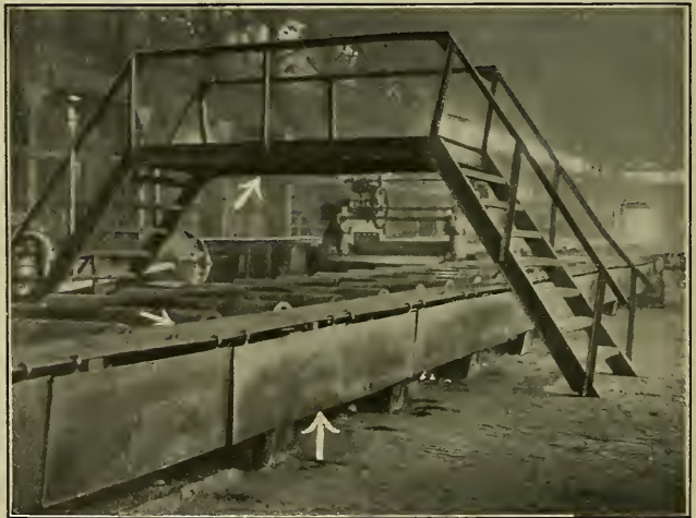
Fig. 43. Live Roll Guards and Bridge Over Rolls.
