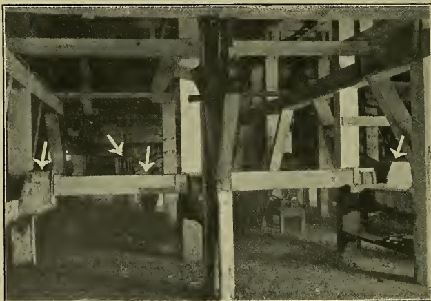
Fig. 47. Guarded Transmission.
