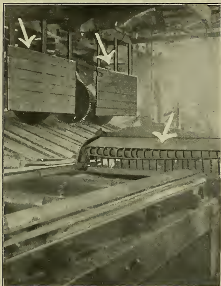
Fig. 19. Finger Guards for Edger.
