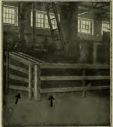
Fig. 294. Slat Belt and Pulley Guards.
