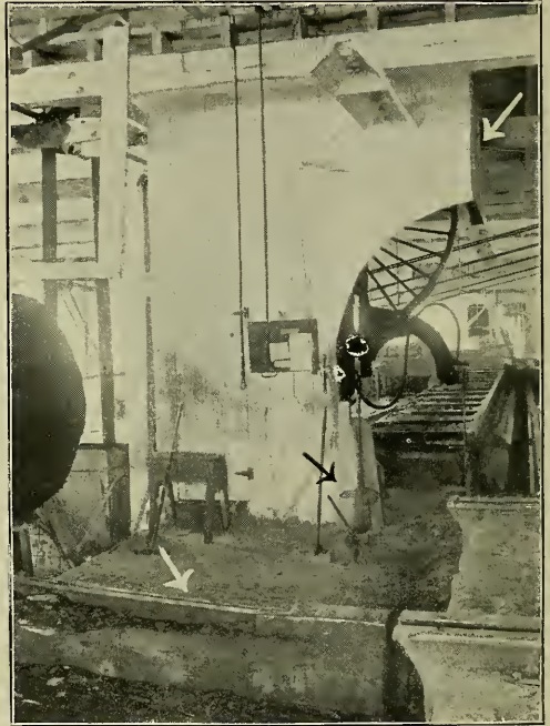
Fig. 9. Deck with Railroad Iron Skids, Band Mill Housing and Lever Lock.
