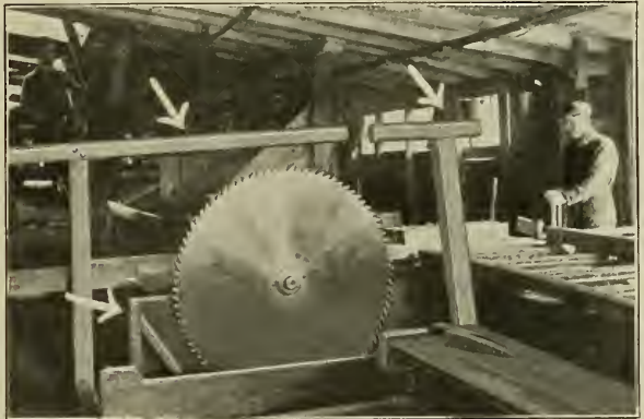
Fig. 67. Shingle Cut-Off Saw Guarded.
