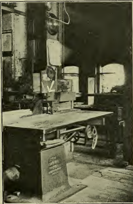
Fig. 261. Grooving Saw Guarded.
