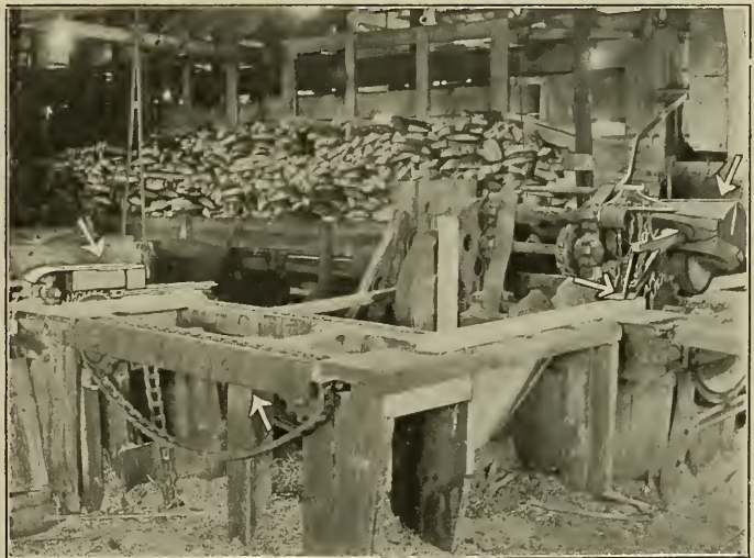
Fig. 60. Lath Bolter and Saws Guarded.
