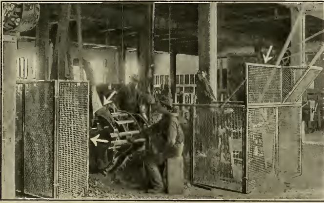
Fig. 217. Spoke Tenoner Guarded.
