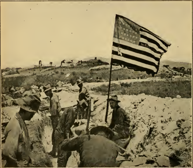
In the Trenches before Santiago
