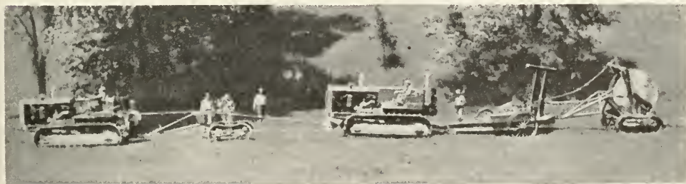
FIG. 16. PLOWING TELEPHONE CABLE UNDERGROUND
