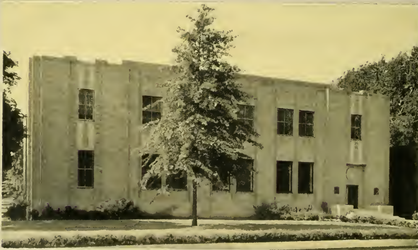
OTTAWA, ONT., CANADA E. I. BAROTT AND F. J. MACNAB, Architects CLEVELAND, OHIO, LAKEWOOD EDWARD G. CONRAD, Architect
