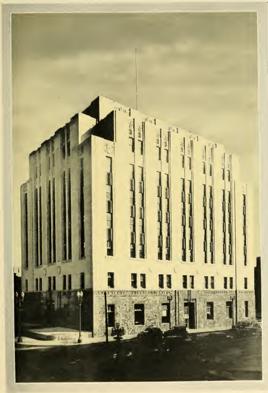
ST. PAUL, MINN., DOWNTOWN C. H. JOHNSTON, Architect
