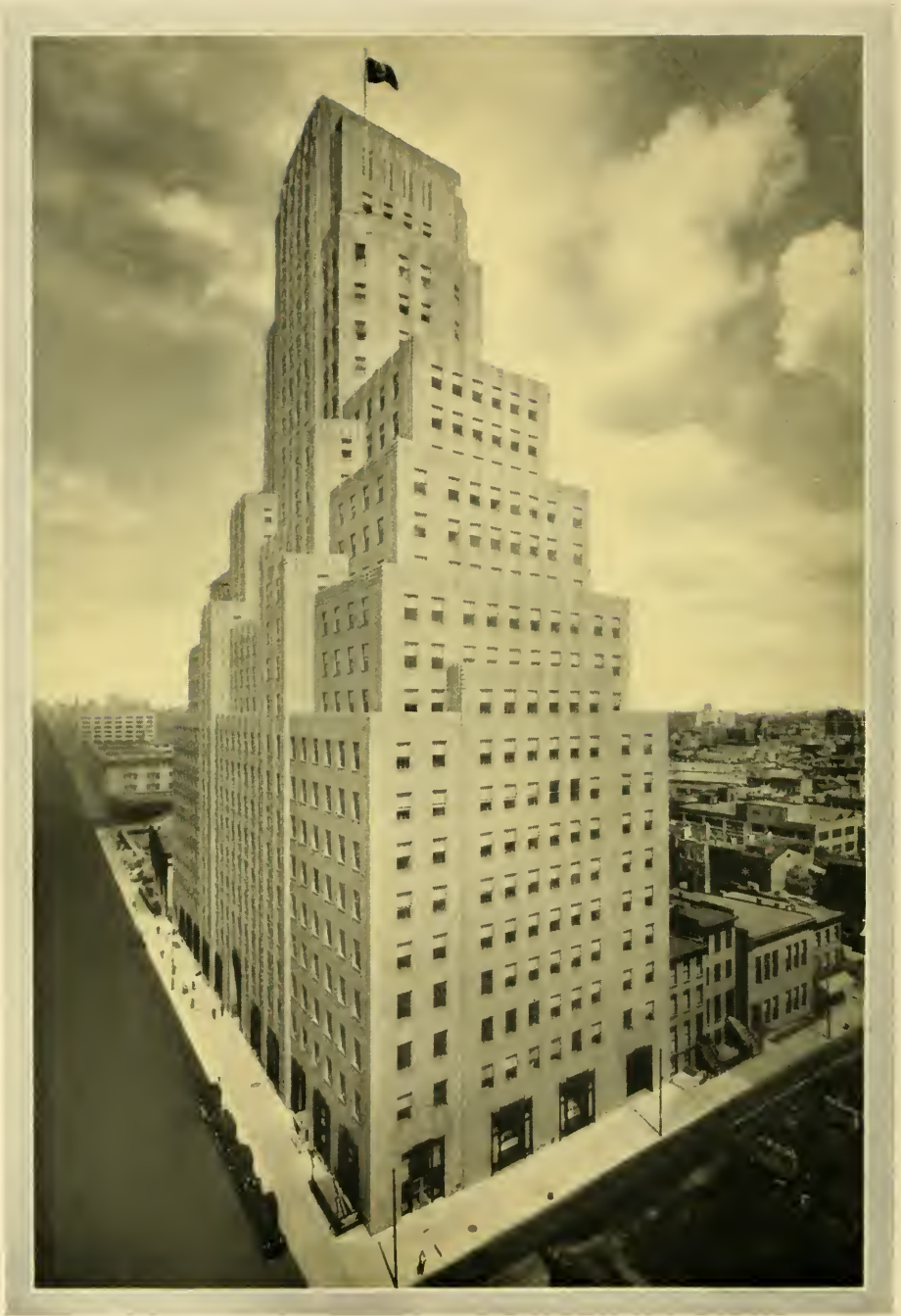
BROOKLYN, N. Y., ADMINISTRATION VOORHEES, GMEIN & WALKER, Architects
