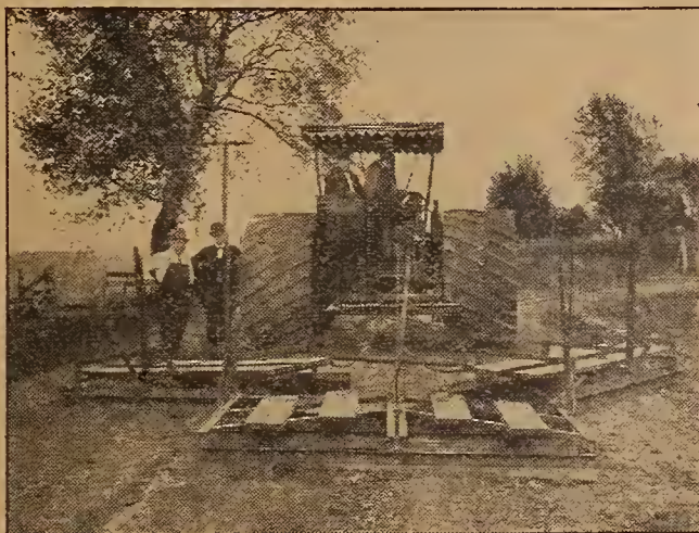
Fig. 2—The three-way drag covers the entire road
