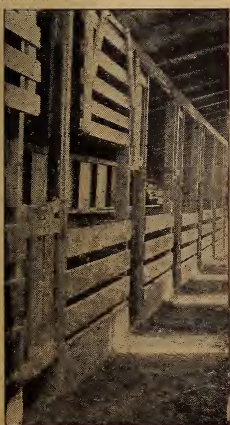
Interior of hog-house showing the adjustable gates
