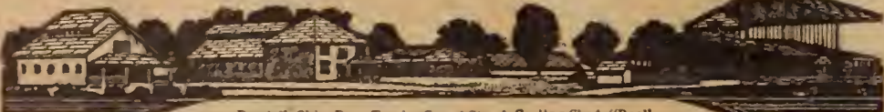
Randall, Ohio, Race Track. Grand Stand, Cooling Shed, "Doc" Watterson's Barn, Sanders' Stables, and all new buildings around Track covered with J-M Asbestos Roofing
