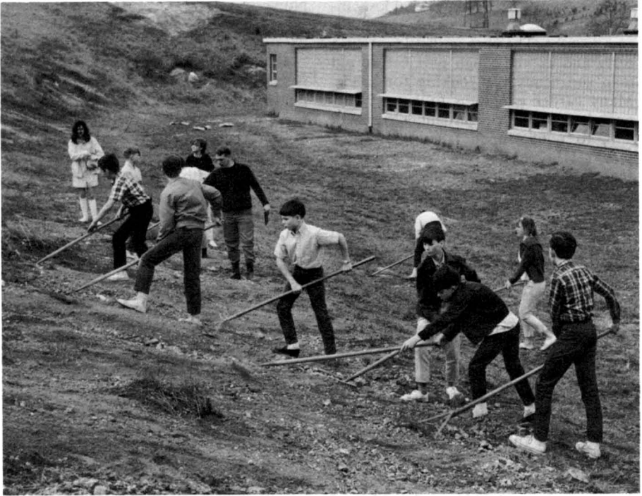
Learning to control soil erosion on a Tennessee school site means shaping and seeding the slope to appropriate grass seed mixtures to protect the soil from water runoff.
