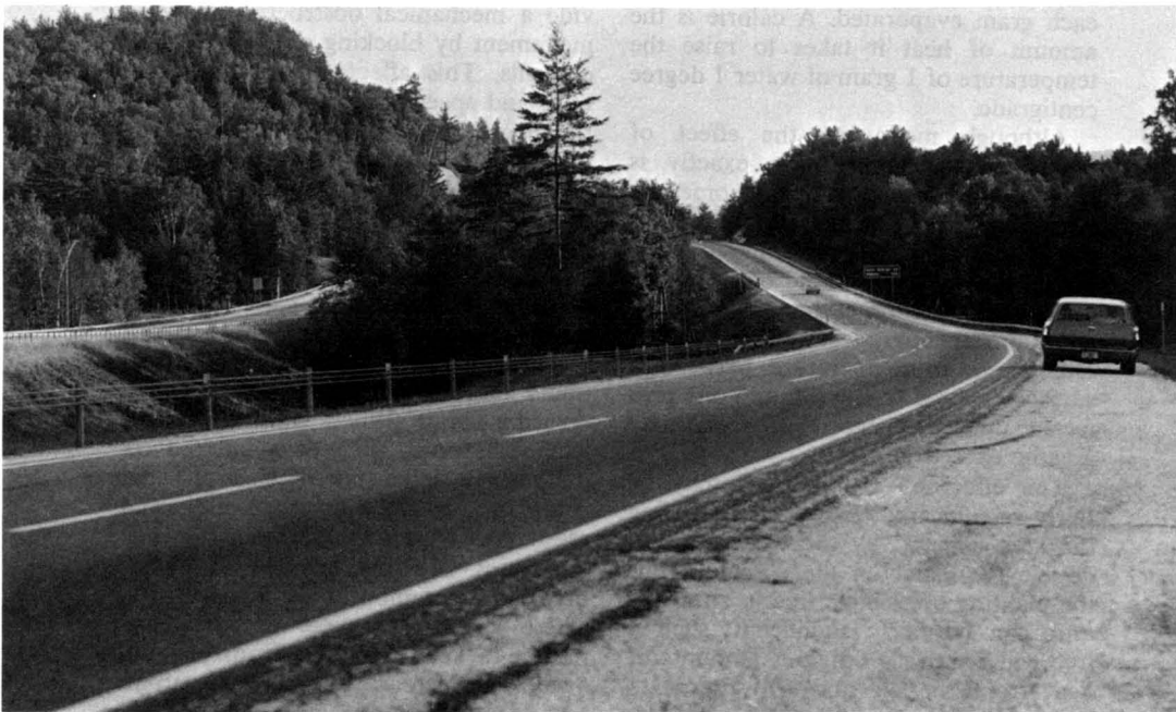
Trees between north and south lanes on this freeway in New York State reduce wind and dust activity, and lower the noise levels, as well as creating a scenic drive.
